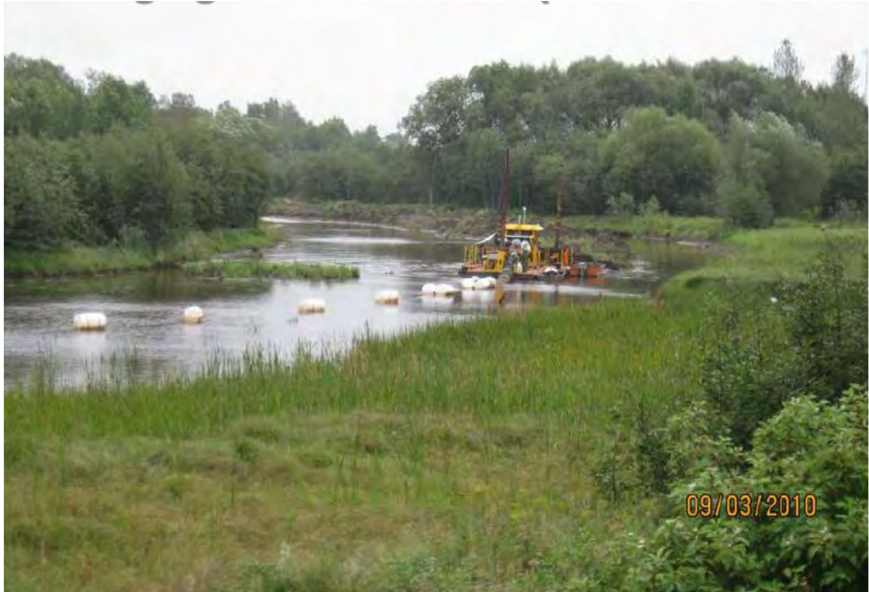
Figure 4. 2010 Dredging of Tallas Bay Underway.
