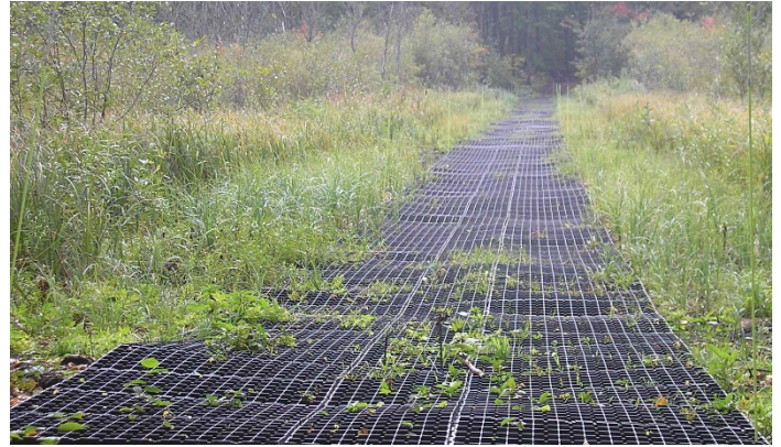
Grass pavers installed on trail tread in Aitkin
