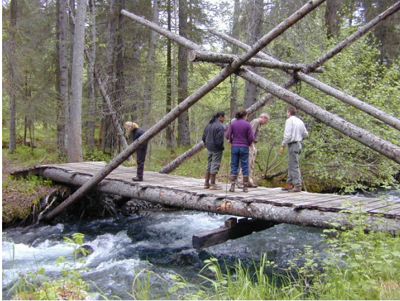
Temporary bridge in Oregon
