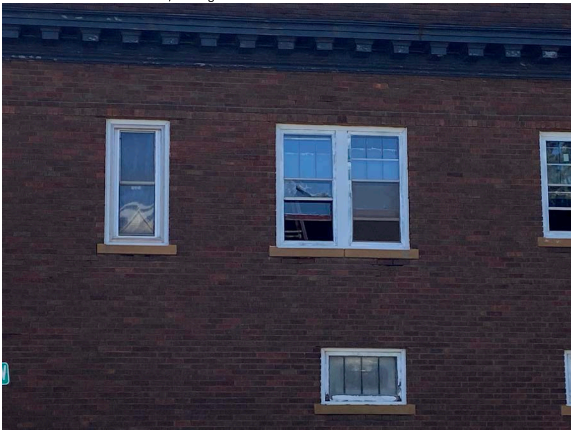
E.45 Windows at east elevation, looking west. Non-historic window at level two is at left side of photo.
