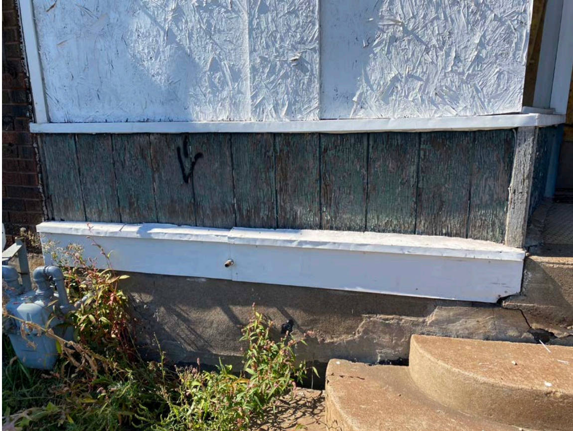
E.42 View of storefront bulkhead and infill panel at west side of first level storefront, looking north.
