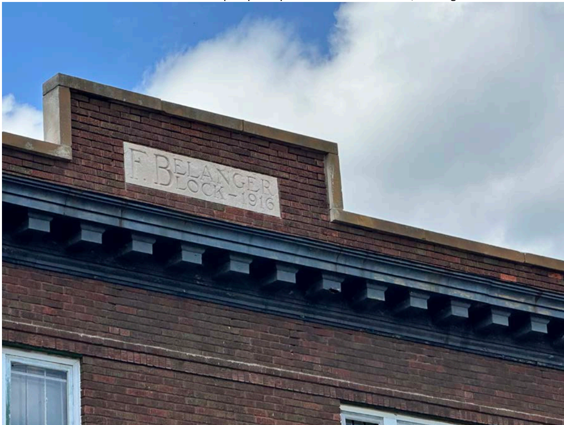
E.33 View of metal cornice and stone parapet caps at the south elevation, looking northeast.
