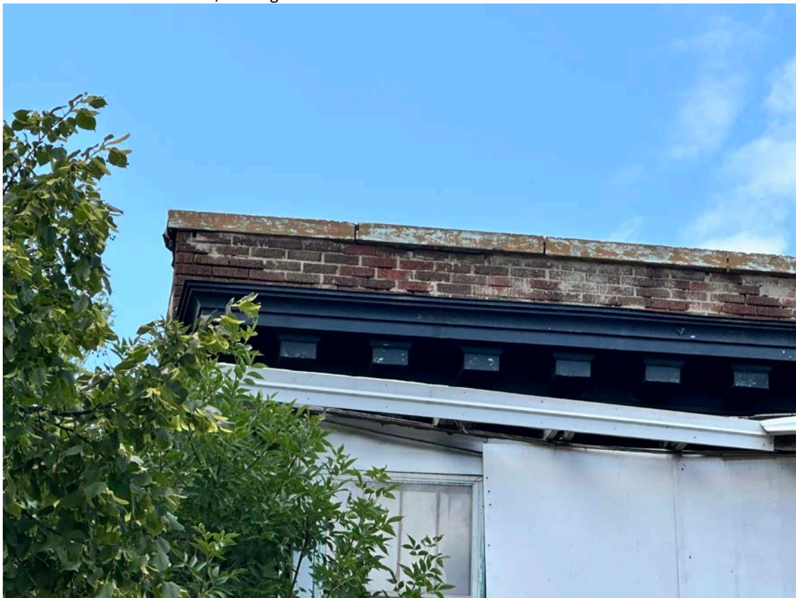
E.31 View of metal cornice and stone parapet caps at the south elevation, looking north.
