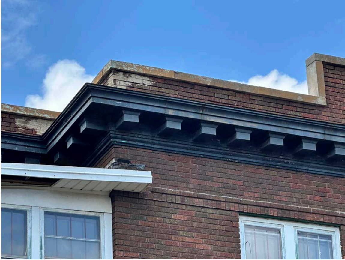
E.32 View of metal cornice and stone parapet caps at the south elevation, looking northeast.
