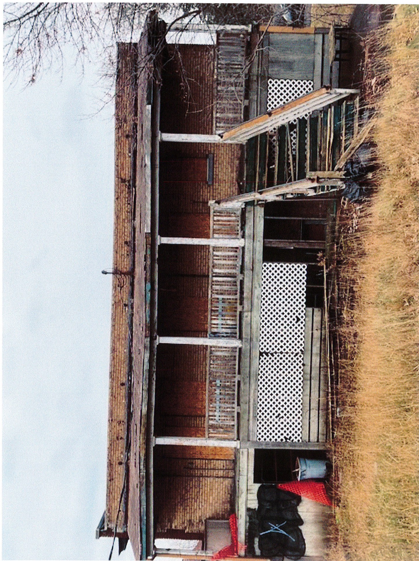
Photo 8: Rear Elevation Showing Dilapidated Original Porch and Stairs
