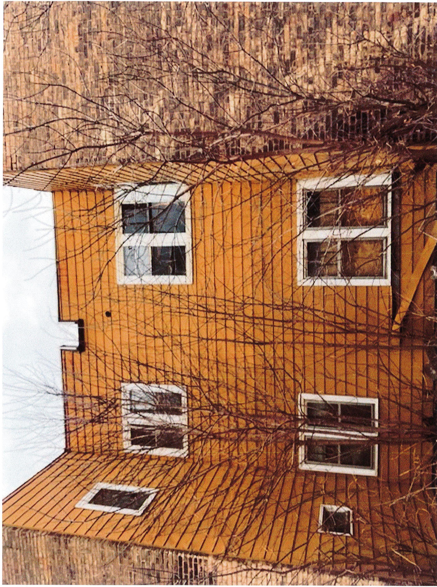
Photo 10: Side Elevation Detail: Recessed Area With Metal Siding
