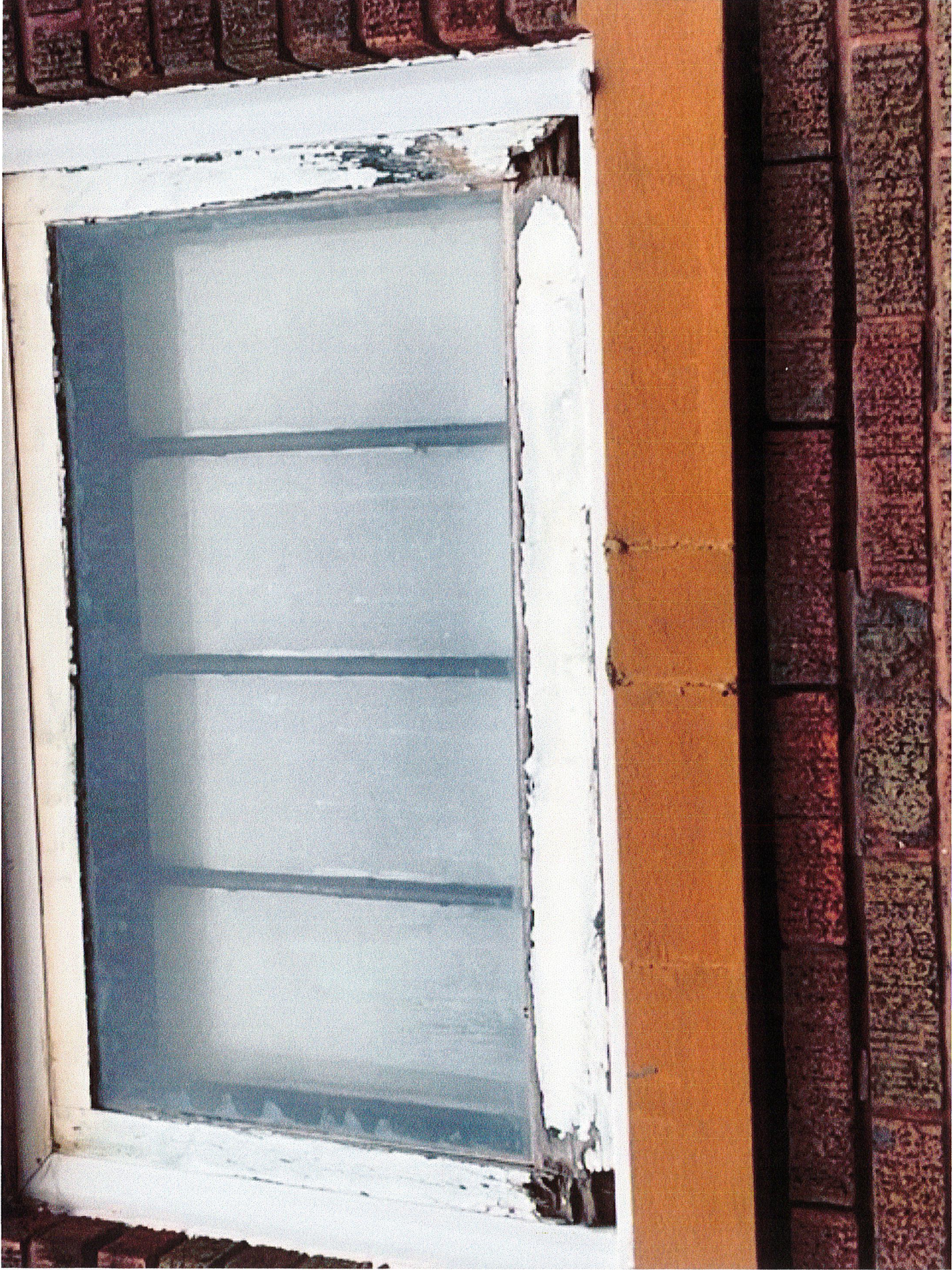
Photo 12: Avenue Elevation Detail: Bottom Rail Rot in clerestory Window #1
