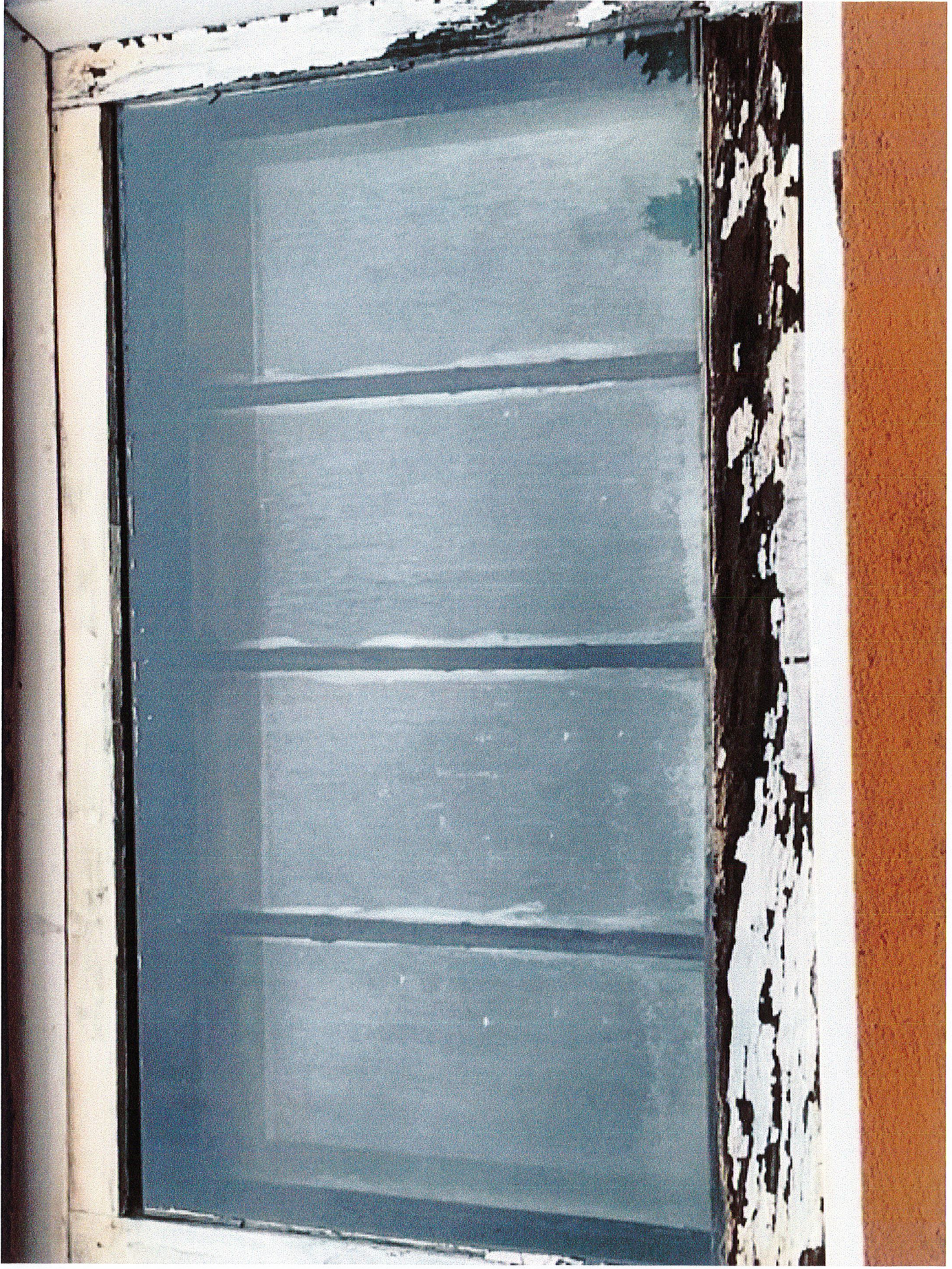
Photo 13: Avenue Elevation Detail: Bottom Rail Rot in Clerestory Window #2
