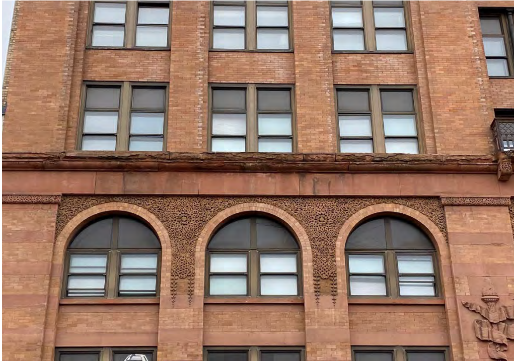
E.47 View of masonry at the south façade of the Board of Trade building, looking north. September, 2022.
