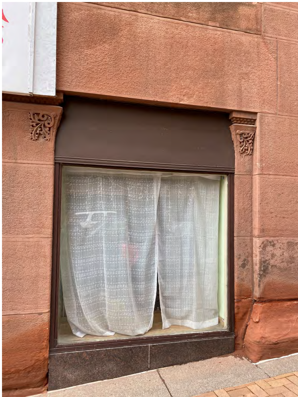
E.54 View of a ground level storefront on the east façade (third from south), looking west. September 2022.
