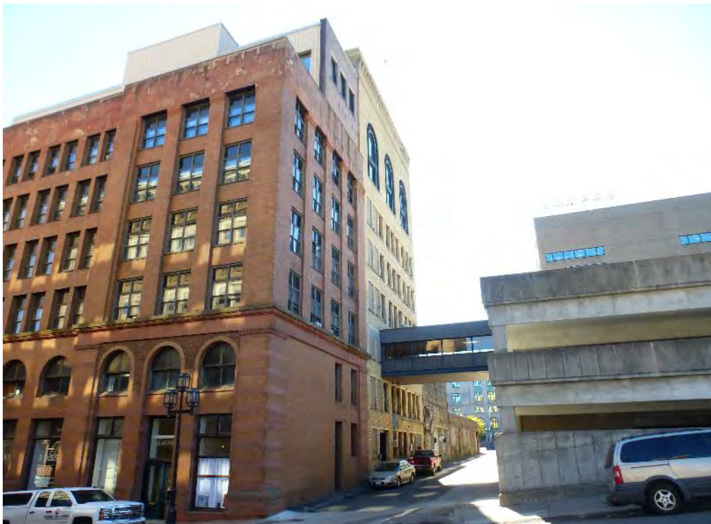
E.11 View of the northeast and northwest façades, looking southwest down the alley. October 2016.
