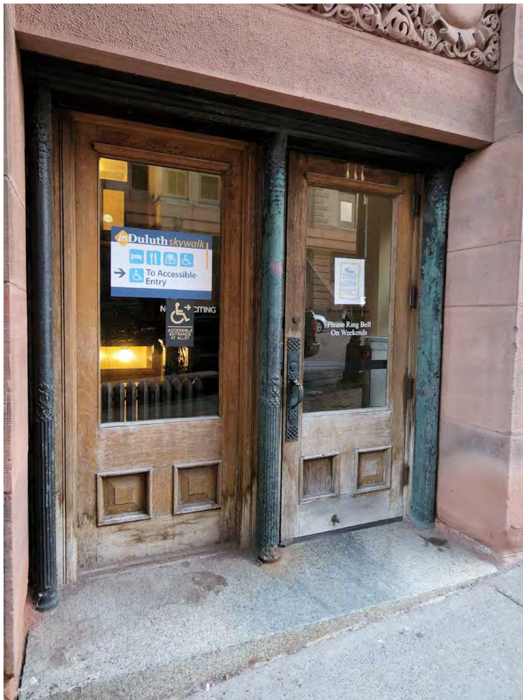
E.59 East façade, southernmost pair of entry doors. September, 2022.
