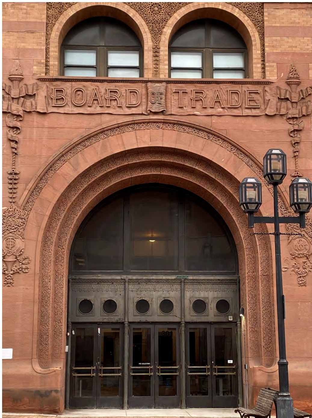
E.50 View of the primary entrance on the south façade, looking north. September 2022.
