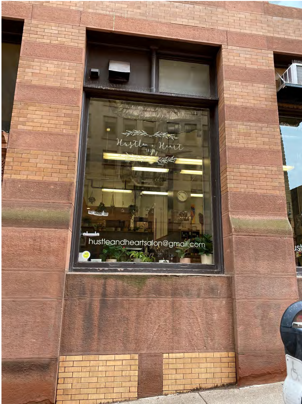
E.60 View of a ground level storefront on the east façade (immediately north of the central entry), looking west. September 2022.
