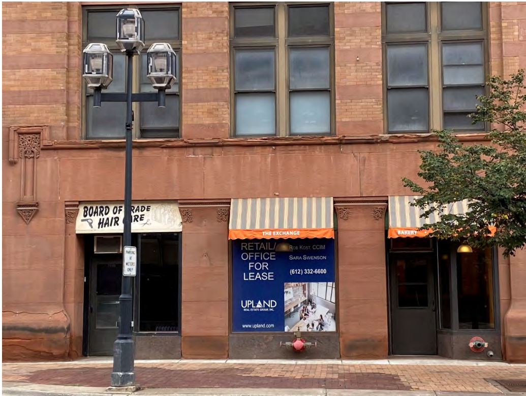
E.49 View of a first level storefront and masonry on the south façade, looking north. September 2022.
