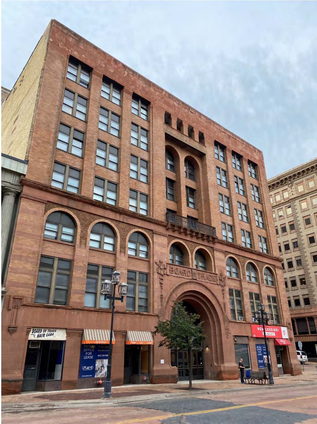
E.46 View of the south façade, looking northwest. September 2022.
