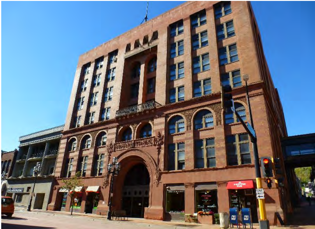
E.03 View of the primary façade (southeast) of the Board of Trade building, looking northwest. October 2016.
