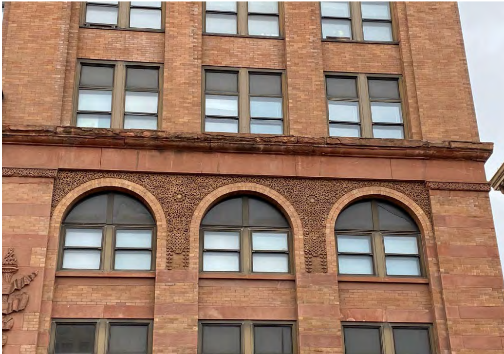
E.48 View of masonry at the south façade of the Board of Trade building, looking north. September, 2022.
