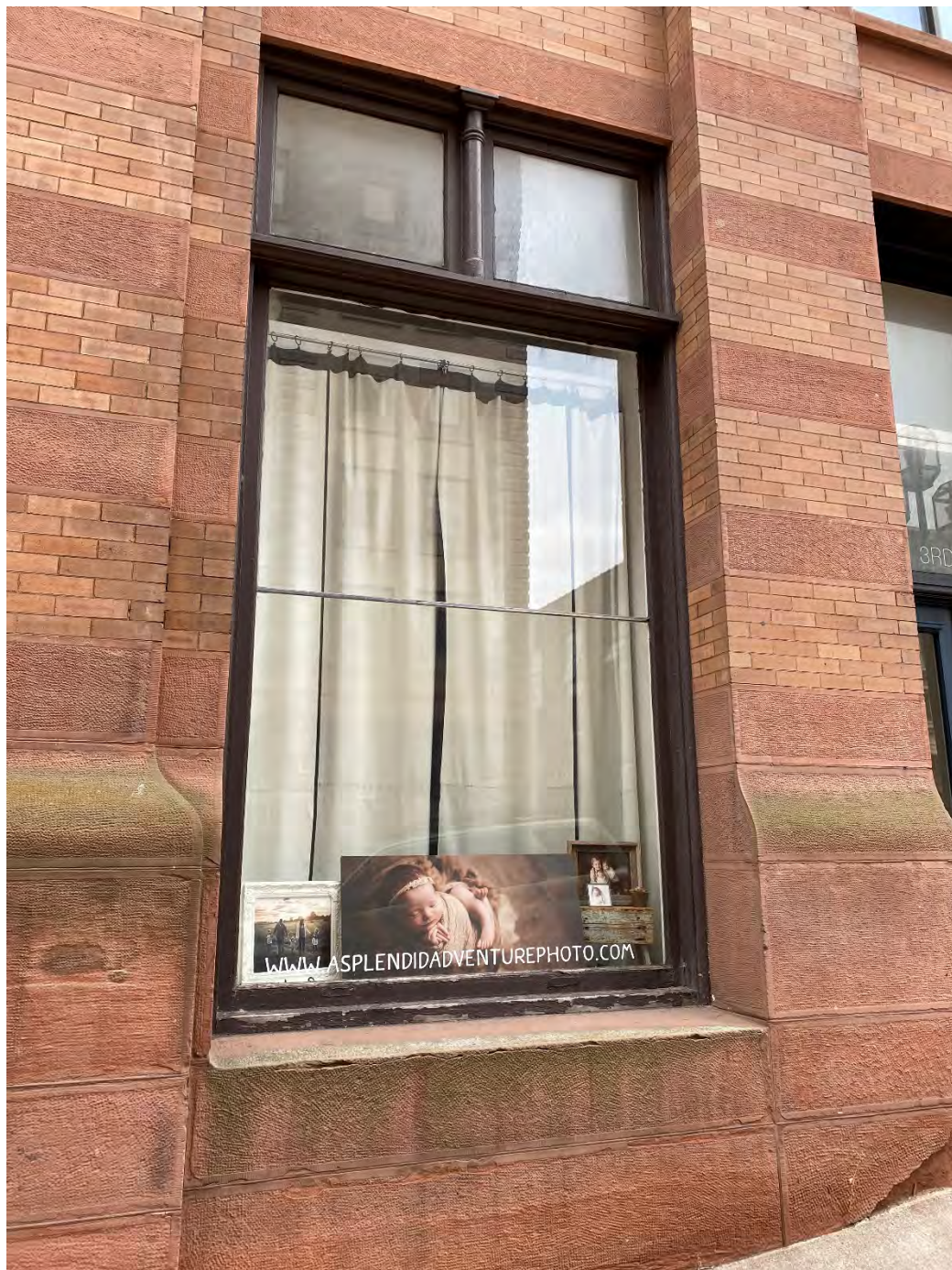
E.62 View of a ground level storefront on the east façade (south of northern entry), looking west. September 2022.
