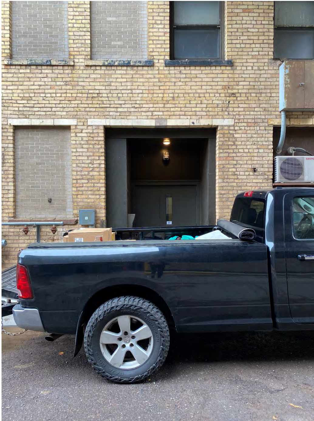
E.65 View of a rear door at the north façade, looking south. September 2022.
