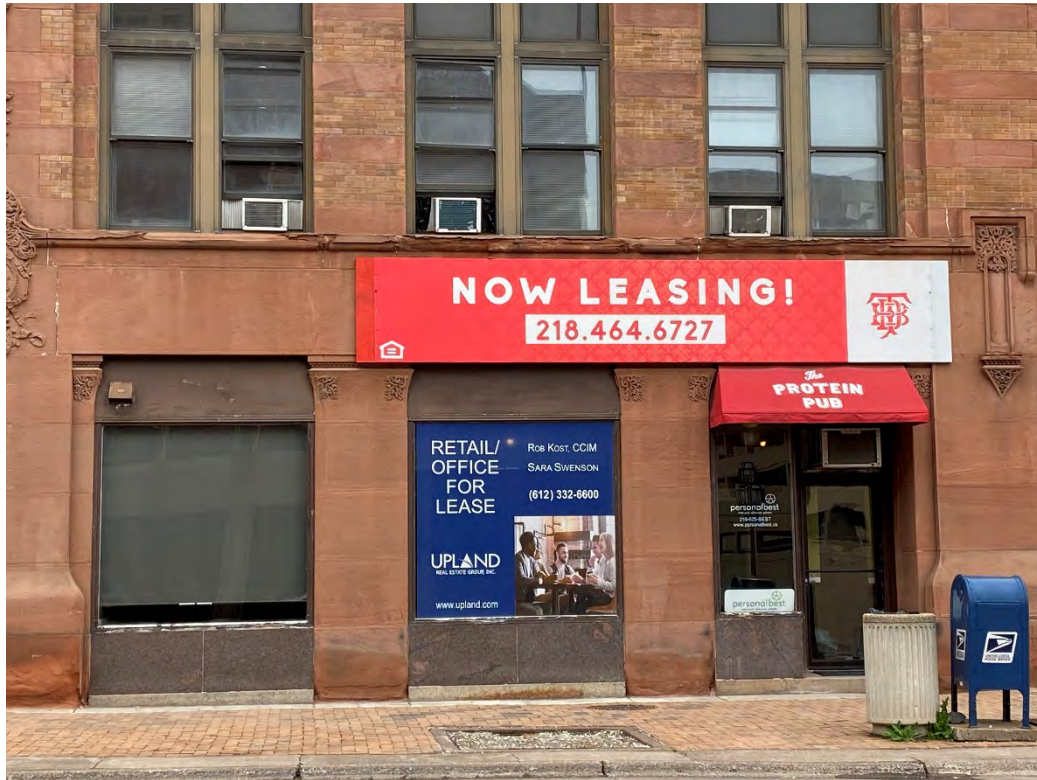
E.51 View of a first level storefront and masonry on the south façade, looking north. September 2022.
