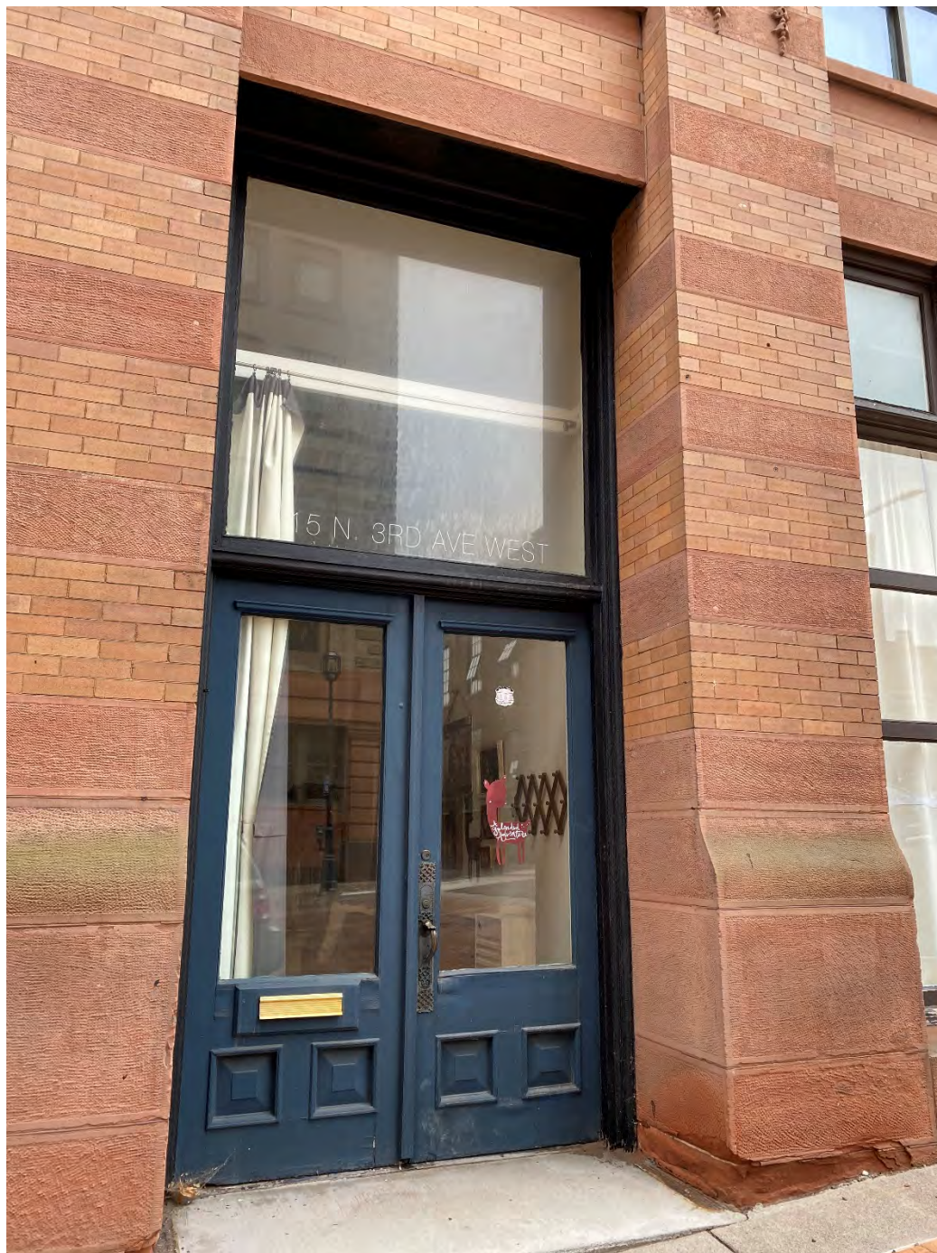
E.63 View of a second level side entry door on the northwest façade, looking southeast. September 2022.
