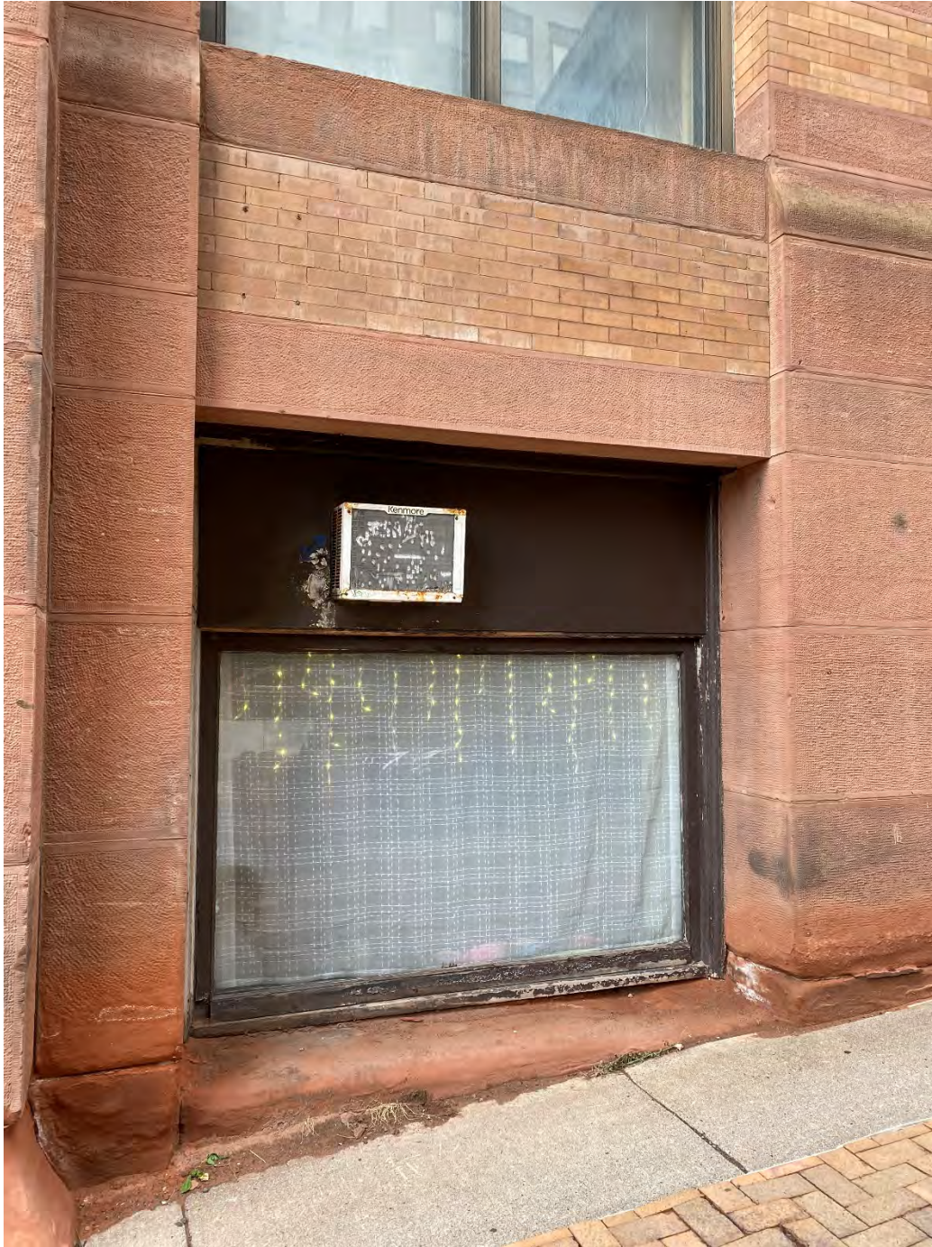
E.55 View of a ground level storefront on the east façade (fourth from south), looking west. September 2022.
