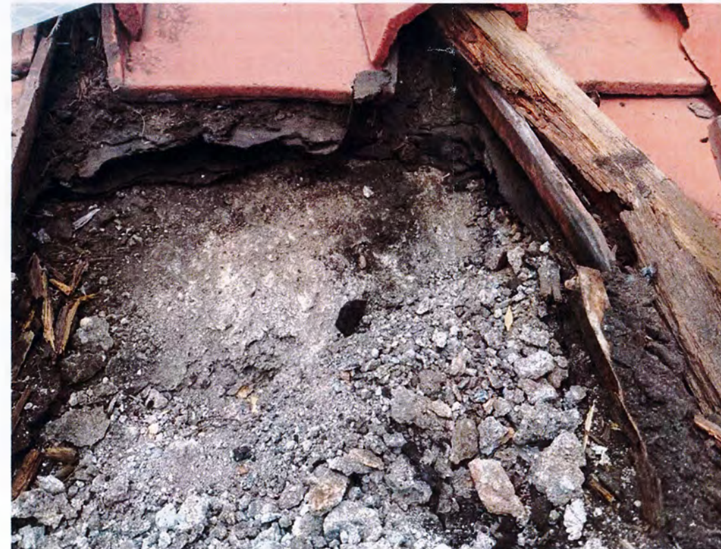
West Slope Demolition Showing Deterioration and Spalled Concrete Roof Deck
