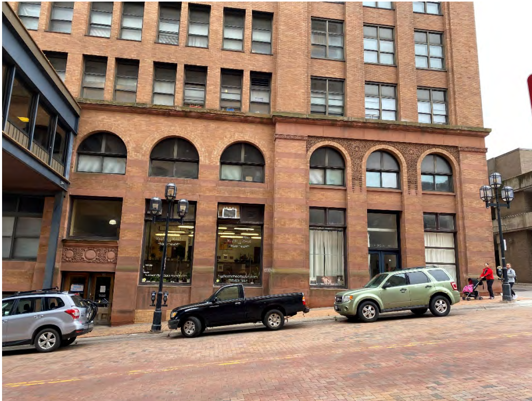
E.58 Northern portion of the east façade, looking west. September 2022.
