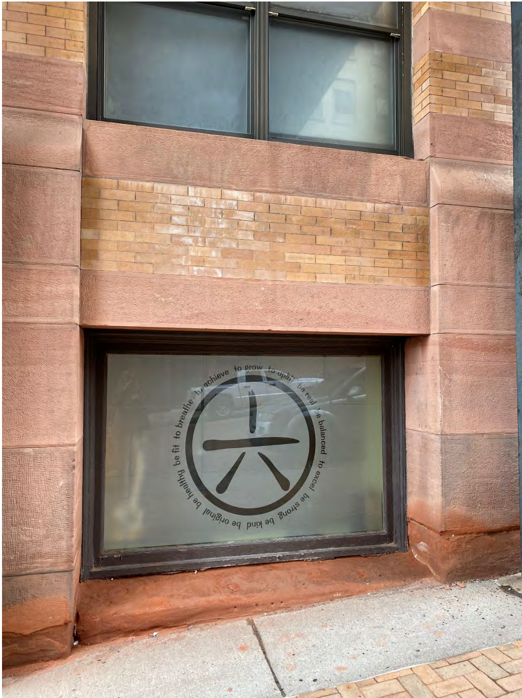
E.57 View of a ground level storefront on the east façade (sixth from south), looking west. September 2022.
