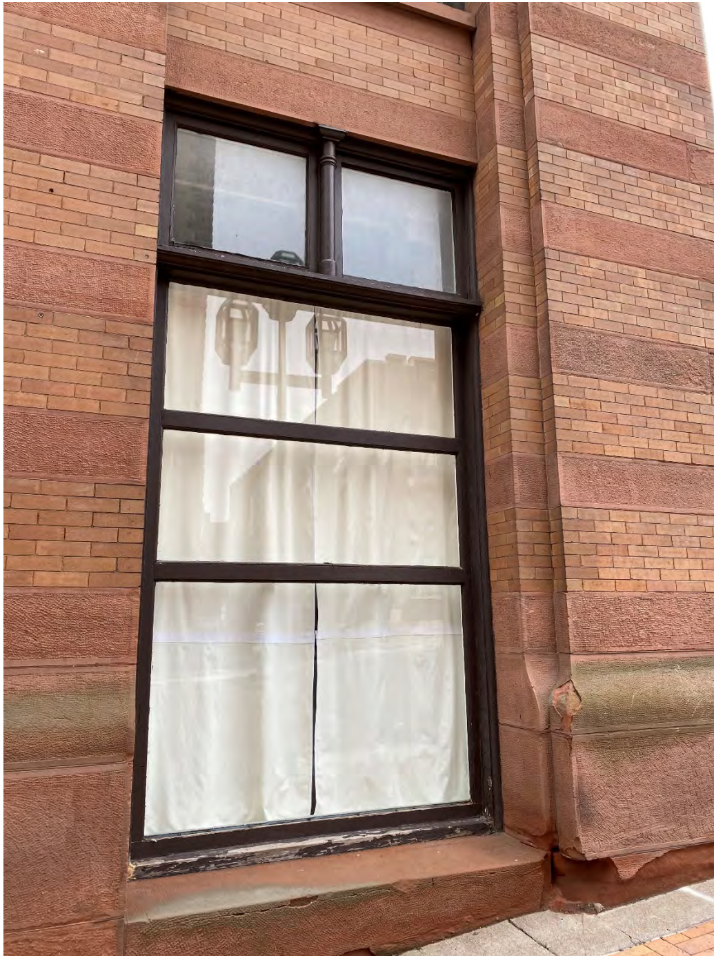
E.64 View of a ground level storefront on the east façade (north of northern entry). September 2022.
