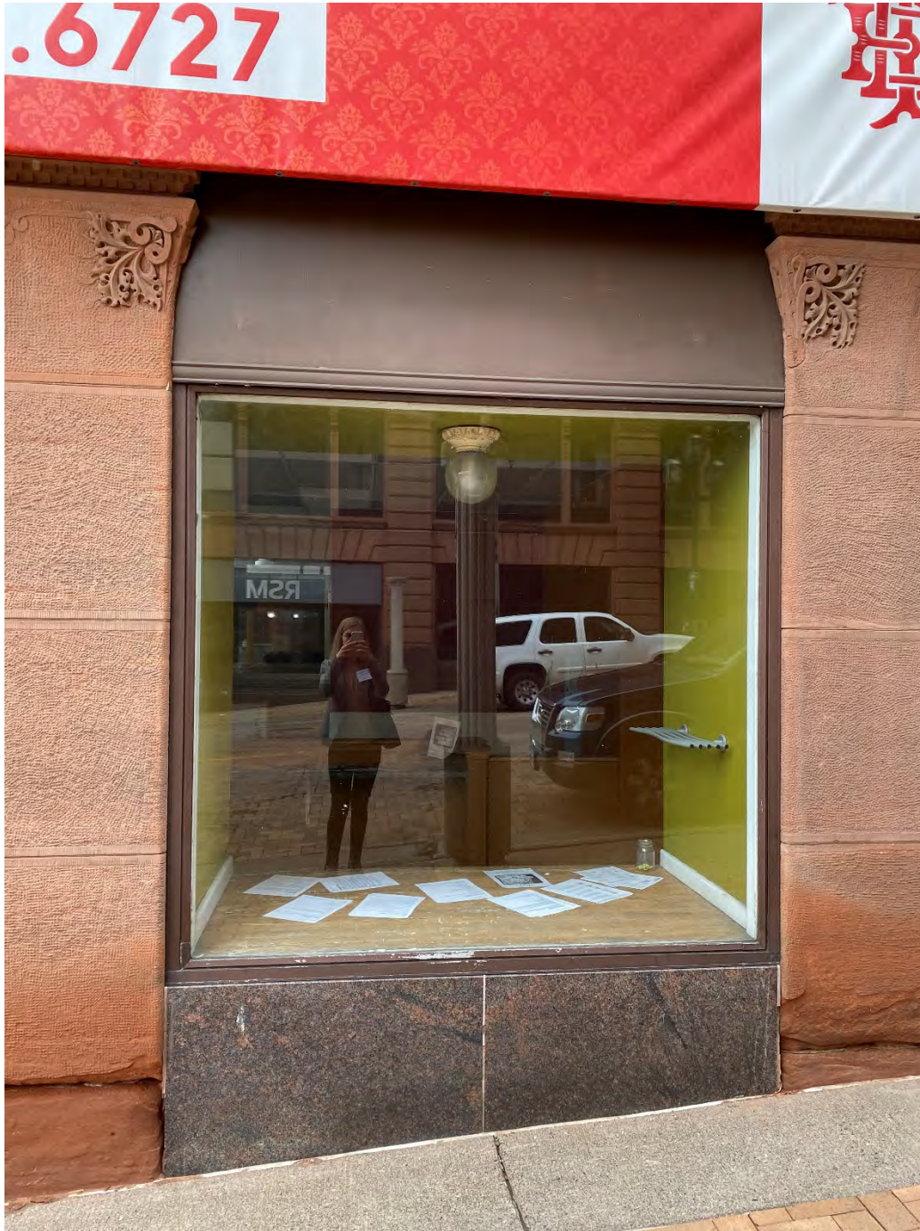
E.53 View of a ground level storefront on the east façade (second from south), looking west. September 2022.
