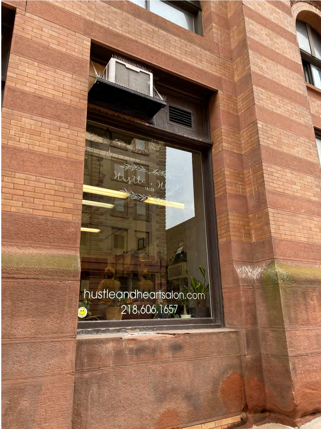
E.61 View of a ground level storefront on the east façade (second to the north of the central entry), looking west. September 2022.
