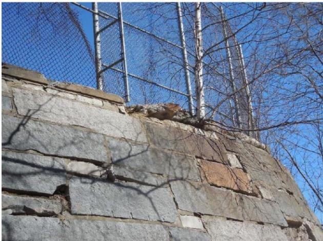
Wall 1, Photo 3: Deteriorated Concrete Cap with Vegetation
