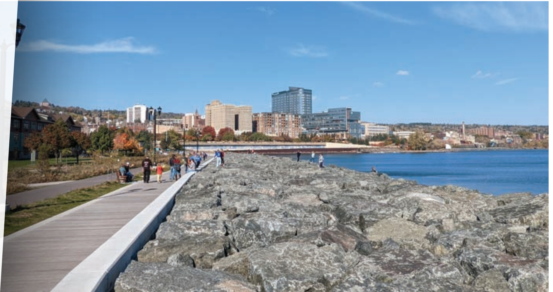
Reconstructed Lakewalk and Coastal Revetment, 2022
