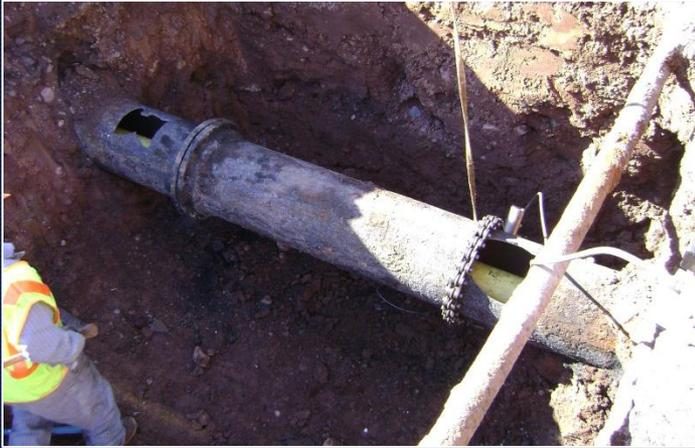
Above: Steel main in cast casing.
