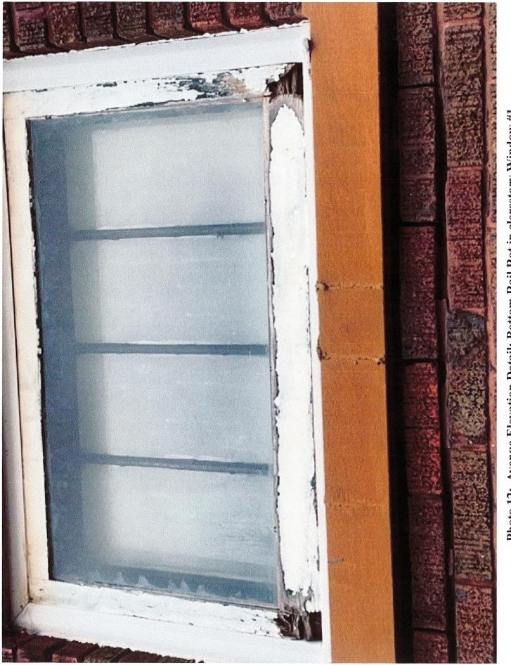
Photo 12: Avenue Elevation Detail: Bottom Rail Rot in clerestory Window #1
