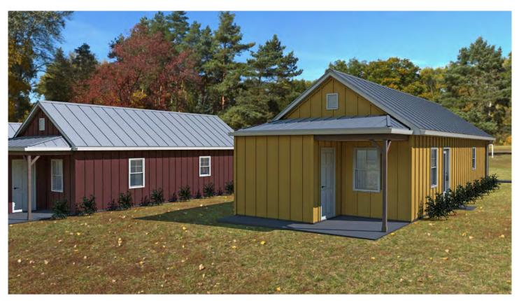
\*Pictured are artistic renderings only. Actual structure will have a 12" heel truss which will make the roof taller above the walls giving the roof a more substantial look.
