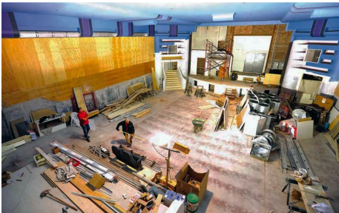
CAPTION: Workers renovating the 1937 West Theater at 317 North Central Avenue. [Image courtesy Duluth News Tribune]
