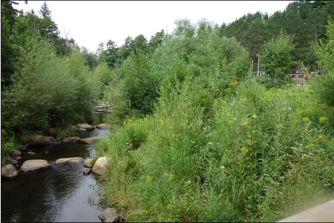
9 (above): Looking northwest on Chester Creek just upstream from where a dam once blocked the flow, creating a lake. The creek was reestablished after the 2012 flood and its banks are filled with vegetation.
