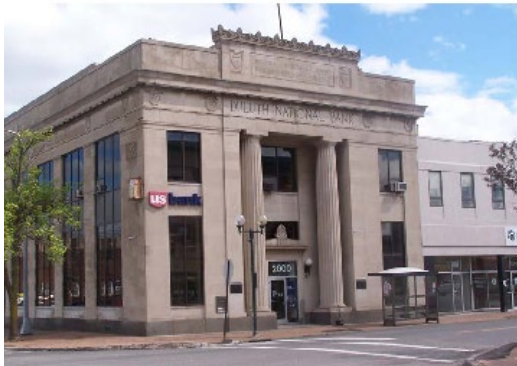
Example of Corridor Building II
