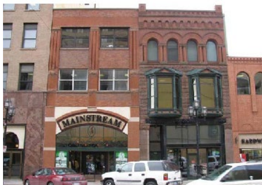
Example of Main Street Building III
