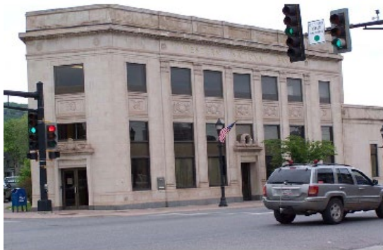
Example of Corridor Building II
