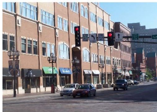
Example of Main Street Building III
