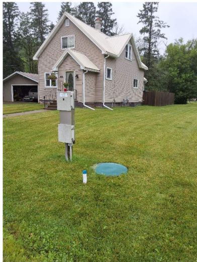
EXTERIOR WORK AREA
