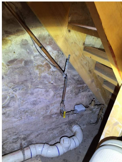
INTERIOR WORK AREA
