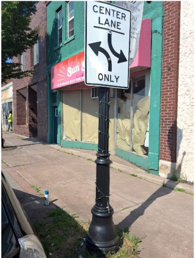
EXTERIOR WORK AREA
