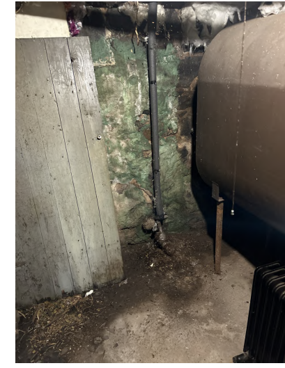
INTERIOR WORK AREA
