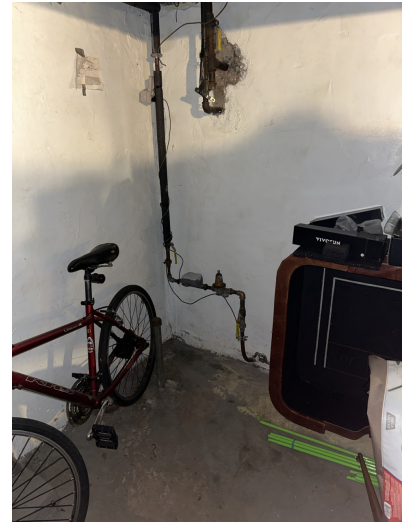
INTERIOR WORK AREA
