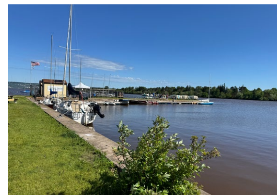
Figure 02.15 Sailing pier with seawall
