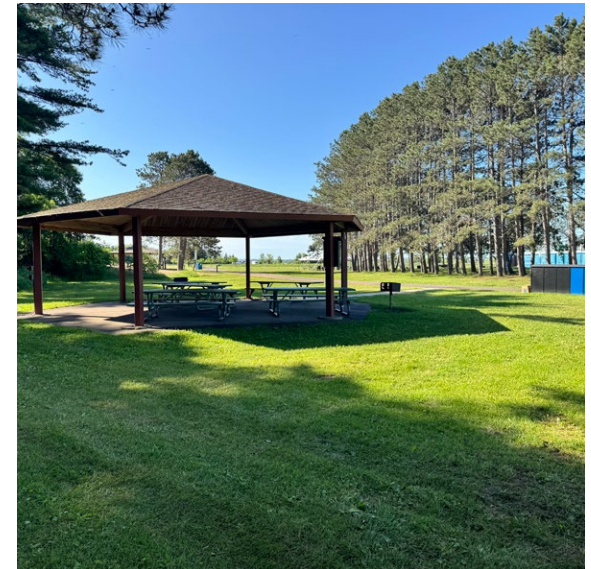
Figure 02.24 Existing picnic shelter
