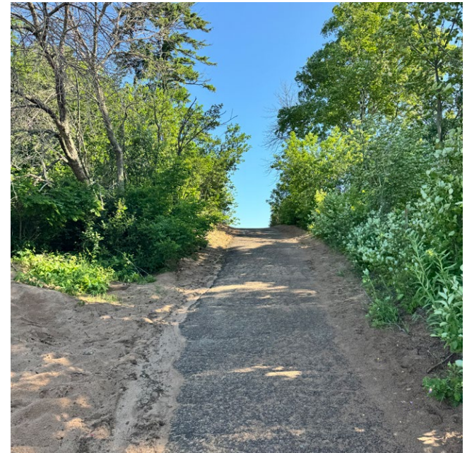
Figure 02.11 Existing maintenance drive (right)
