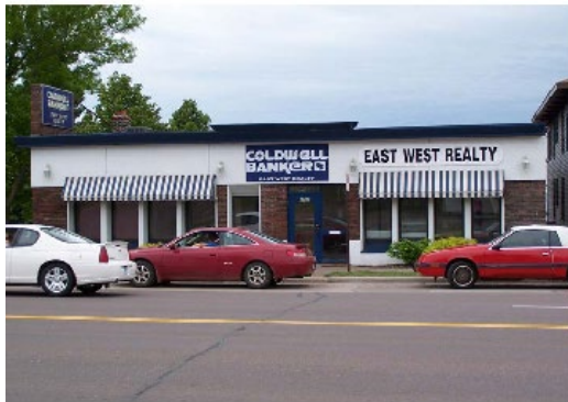
Example of Corridor Building I
