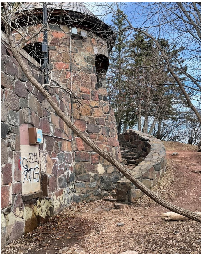
Photo 4: View of east stair from walkway to the lake.
