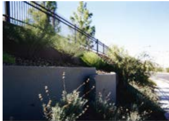
Figure 50-26.4-B: Retaining wall terracing and articulation
