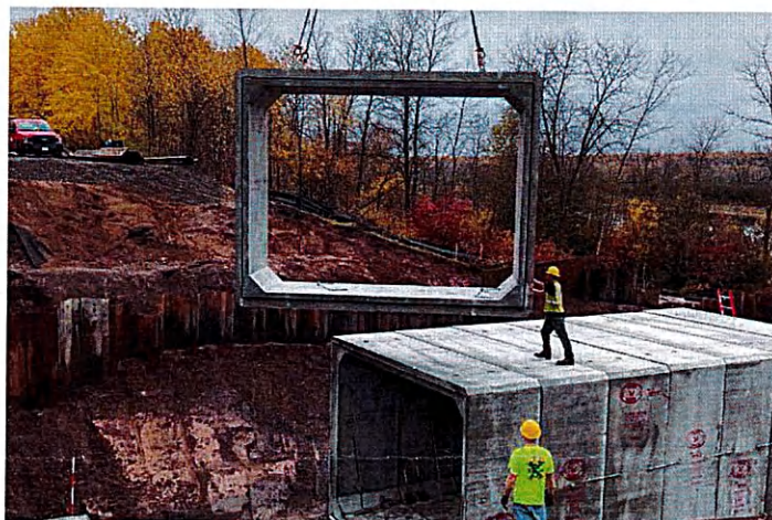
Left Photo: An aerial photograph of Perch Lake after dredging and hemi-marsh construction. The Highway 23 causeway and City-owned trail causeway are adjacent to each other and to the right of this photograph. Right Photo: The installation of the culvert under Highway 23.
