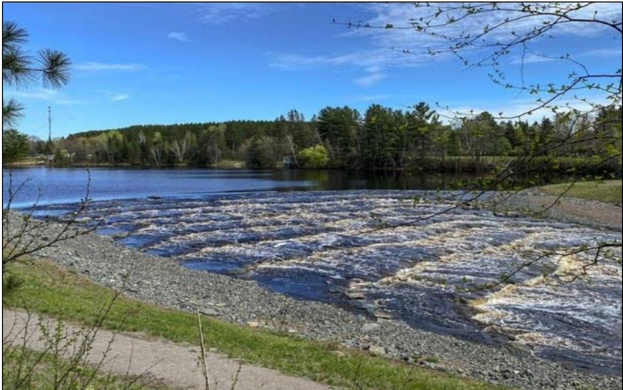
Figure 9: A rock arch rapids on the Willow River in Pine County, MN. Photo courtesy of the MN DNR.
