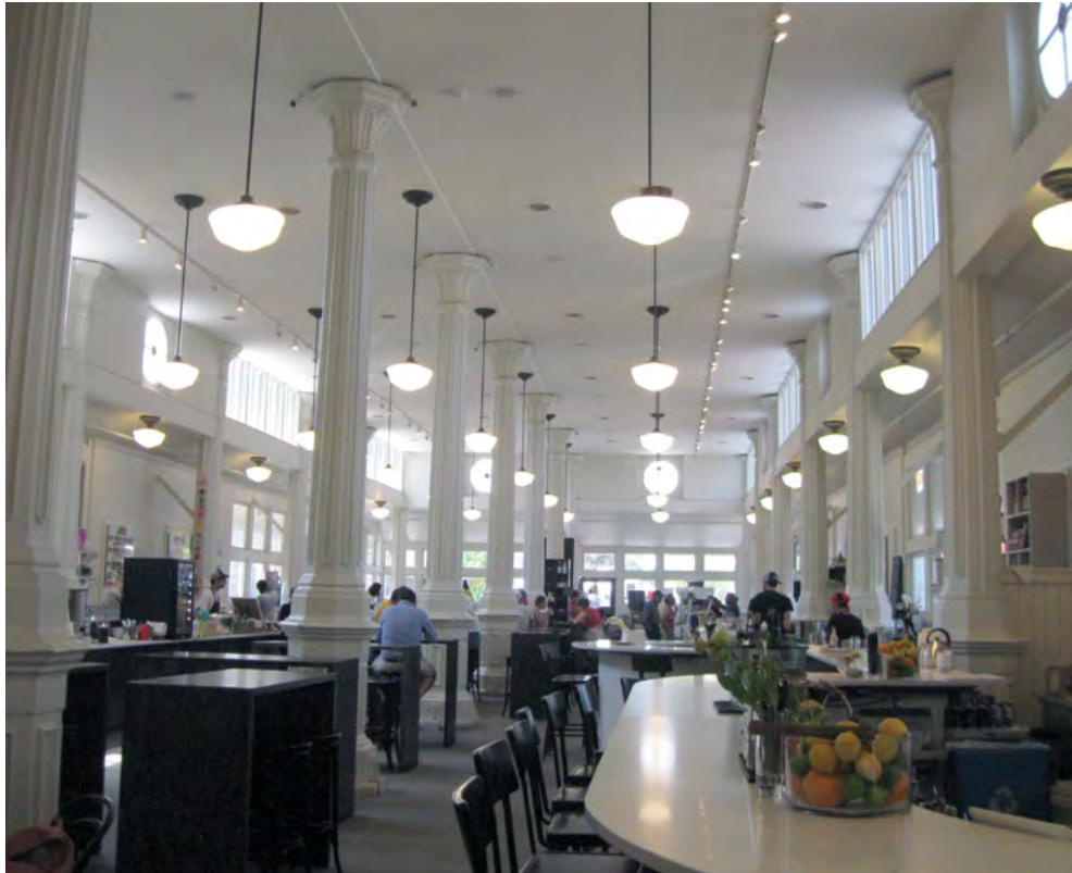
[14] Interior cast-iron columns have been cleaned and repainted as part of the rehabilitation of this historic market building for continuing use.
