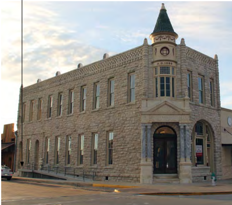
[53] This entrance ramp (right) is compatible with the historic character of this commercial building.
