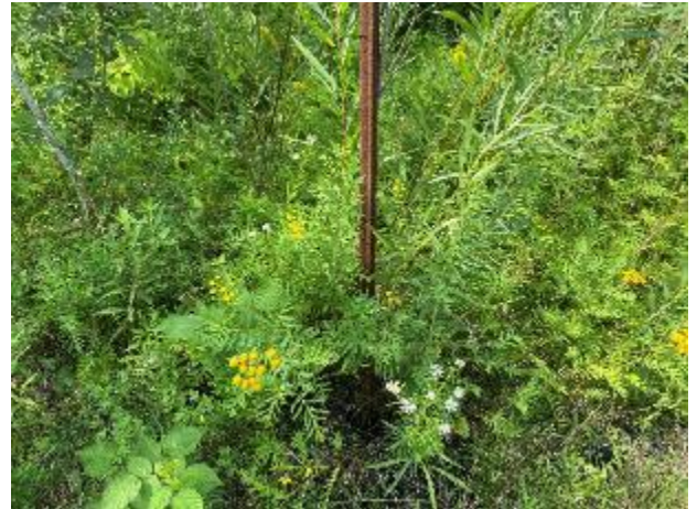
Continued fence post farther south
