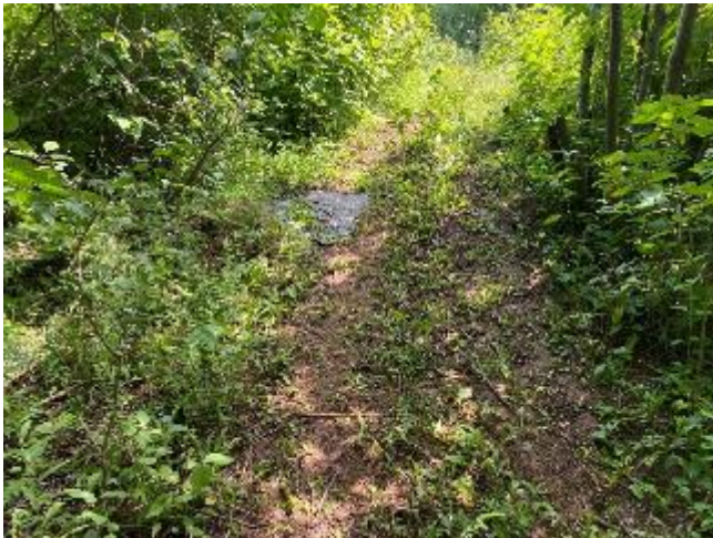
Possible culvert observed along foot trail
