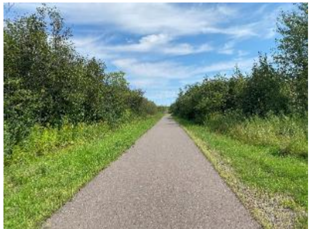
Paved trail facing northeast
