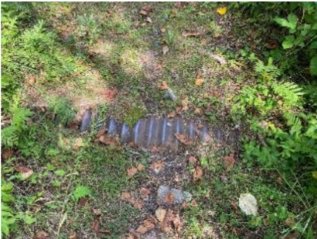
Possible culvert observed along foot trail
