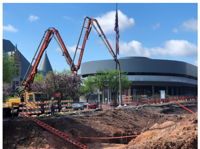
Concrete poured into an old vault in front of the library
