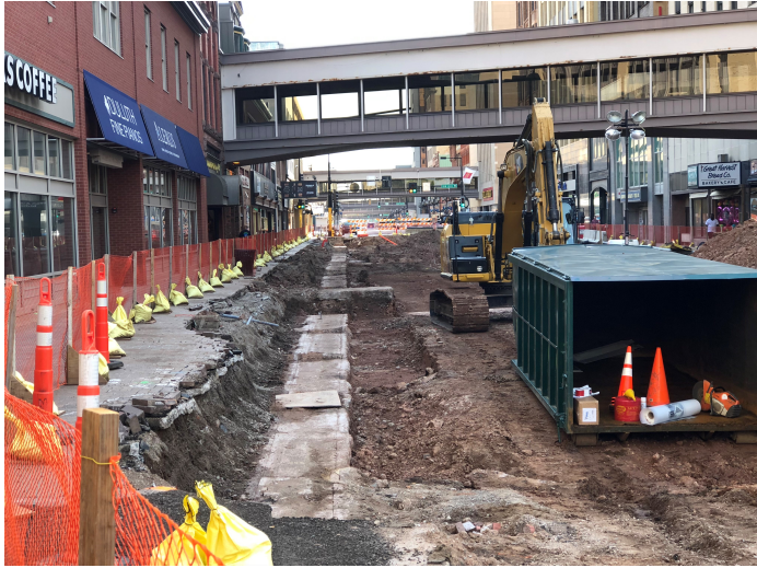
unearthed concrete casing for steam lines
