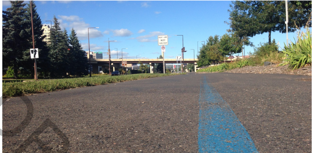
>>Photo Credit: Bikelane Pavement Striping Lakewalk, Jim Shoberg
