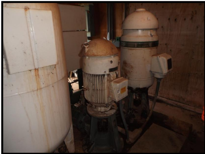
Photo 2: The irrigation pumps at Enger Golf Course are only capable of pumping 850 gpm.
