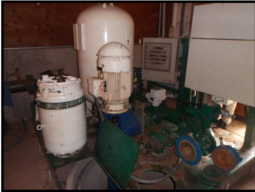
Photo 3: Pump station is undersized and lacks adequate water supply.
