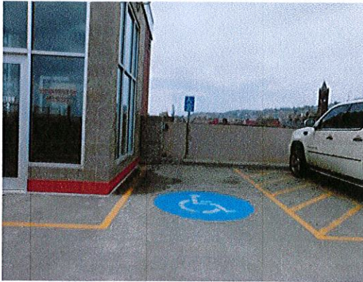
Photo 1: Currently 3 of the parking spaces provide 8' aisles. The other 8' parking spaces have 5' wide aisles. (Complied at time of construction.)
