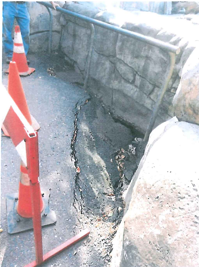
Figure 2: Sidewalk Failure
