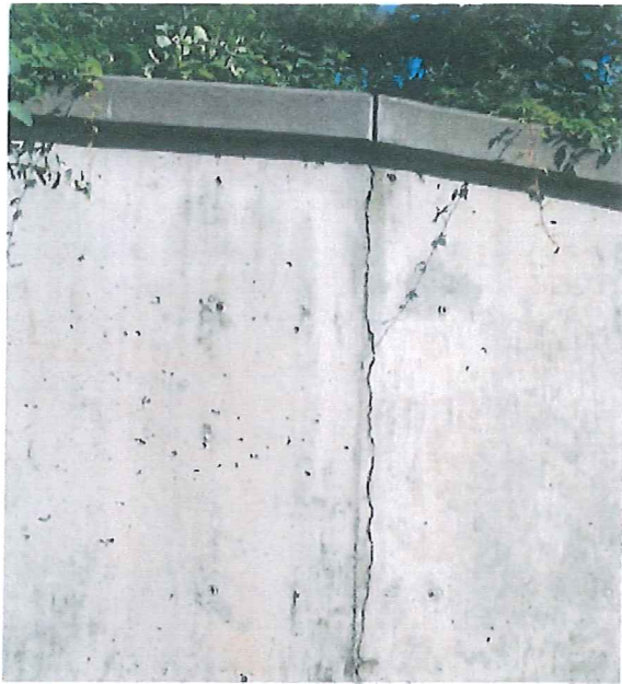
Figure 4 – Vertical cracks in retaining wall
