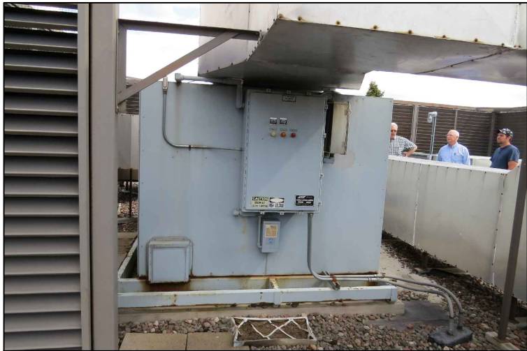
4 EXISTING ROOFTOP DEHUMIDIFIER TO BE REMOVED
