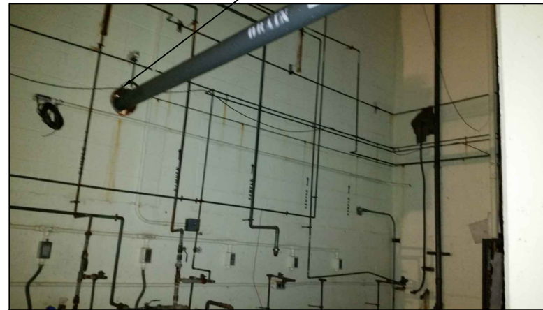
6 SAMPLE PUMP PIPING
