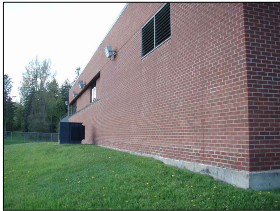
9 WTP WEST WALL
