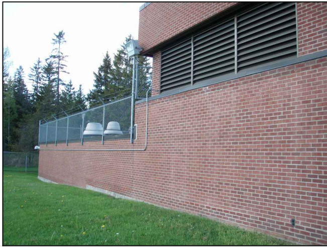
2 WTP WEST WALL
