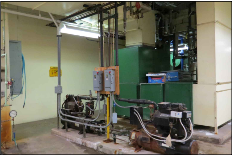
2 EXISTING CONDENSATE PUMPS TO BE DEMOLISHED
