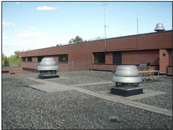
6 WTP LOWER ROOF
