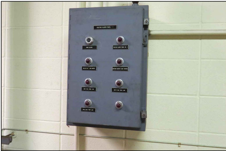
1 EXISTING TEMPERATURE CONTROL PANEL NO.2 TO BE DEMOLISHED
