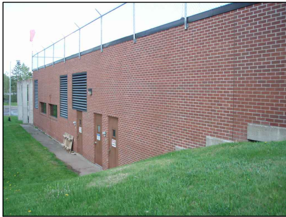
8 WTP NORTH WALL
