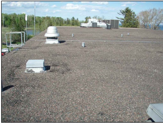
1 WTP UPPER ROOF
