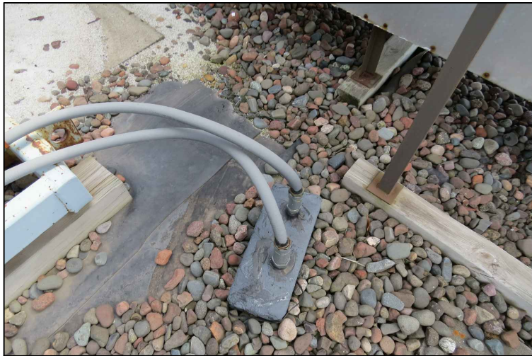
6 ROOFTOP ELECTRICAL CONNECTIONS TO BE ABANDONED
