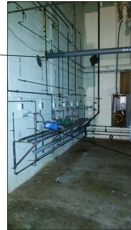
7 SAMPLE PUMP PIPING
