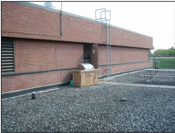
5 WTP LOWER ROOF
