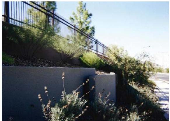
Figure 50-26.4-B: Retaining wall terracing and articulation
