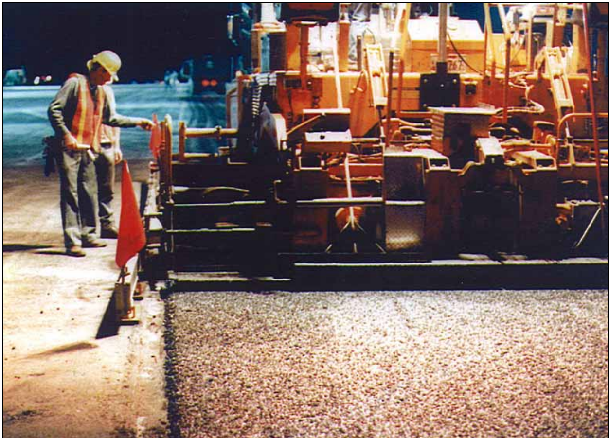
Figure 3. Pavement Spreader in Nighttime Construction
