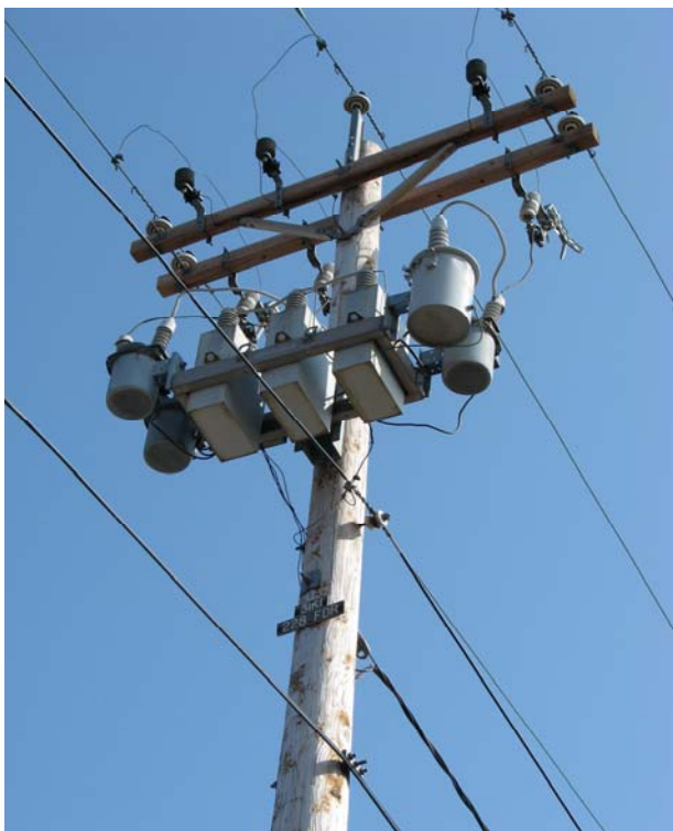
Photo 33 Pole-mounted transformers on southern side of Lot C area. Beside 8th Ave. West alleyway.
