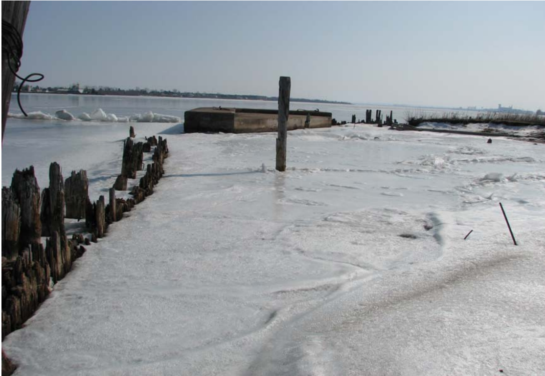
Photo 25 View southeastward toward mouth of Slip 3 (on left). Second eroded area with concrete dock wall moorage element at corner beside mouth of Slip 3.
