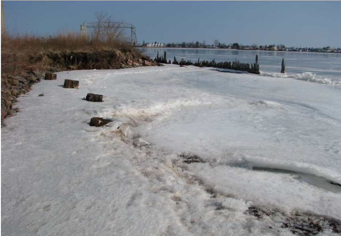
Photo 21 Southeastern side of Lot D area near Slip 3. Portion of filled pier now eroded away. Vertical wood boards mark approximate former dock wall. Fill with debris visible on eroded embankment.
