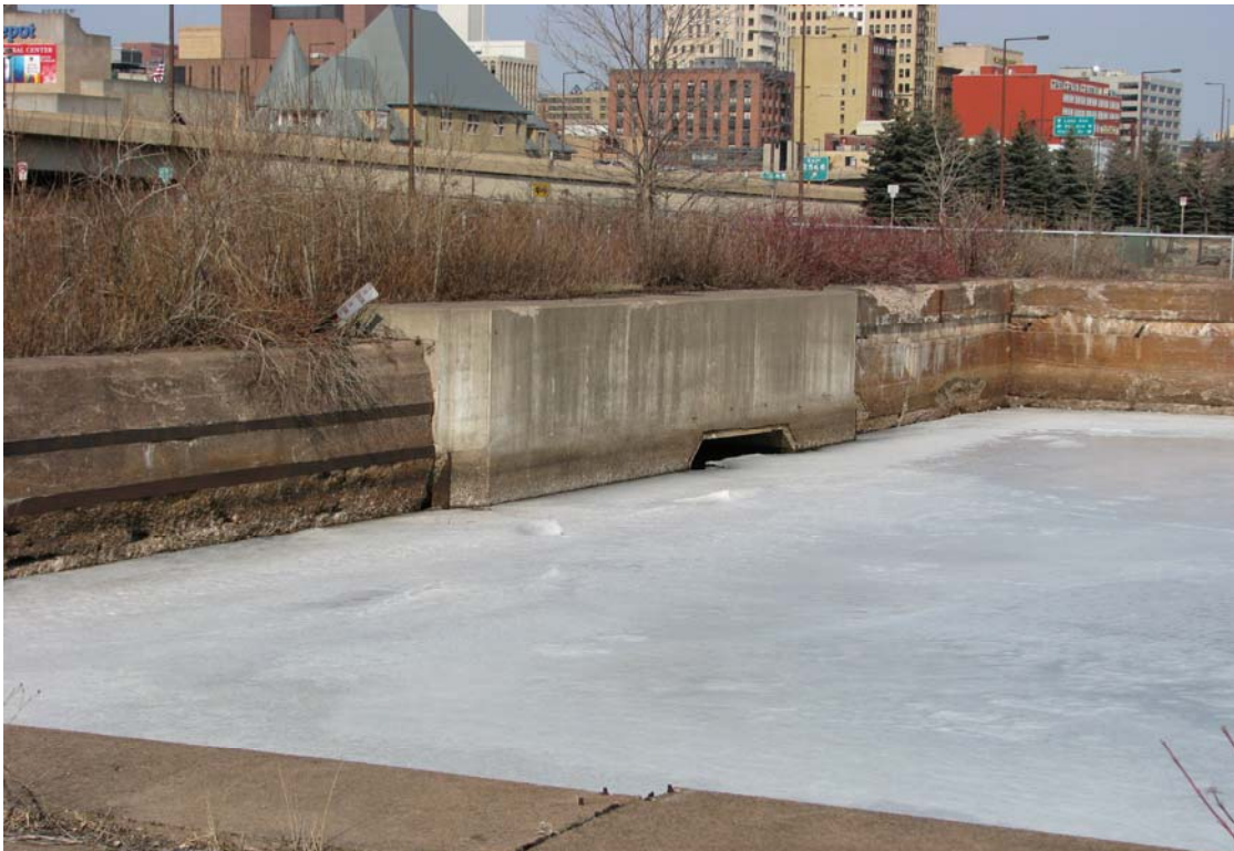
Photo 40 Storm sewer outfall structure at head of Slip 2. Downtown Duluth in background.
