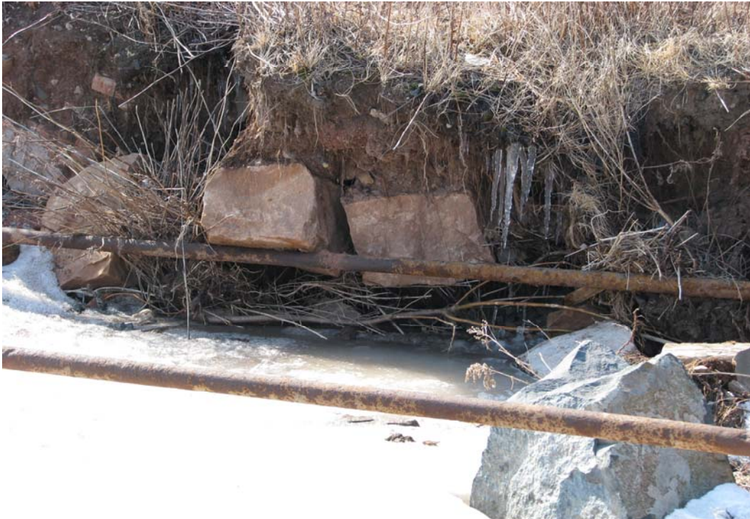
Photo 22 Close-up of steel tie rods, with dimension stone and fill soil displaying filled nature of constructed pier - Lot D area. Photo taken at eroded southeastern side Lot D area.
