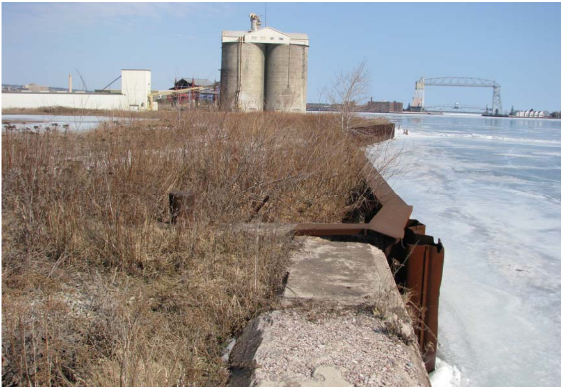
Photo 20 Southeastern side of Lot D area. View northeastward along concrete and steel sheet pile dock wall. LaFarge cement silos in background. Harbor on right.
