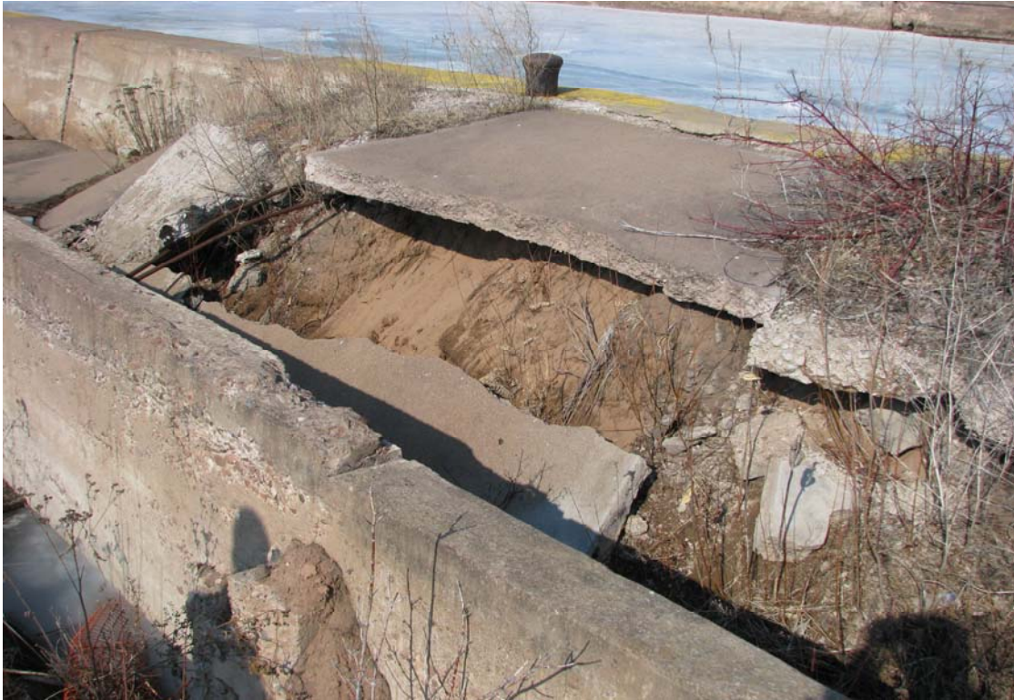
Photo 39 Collapsing section of Slip 2 dock wall structure on Lot C. Sand fill visible beneath cement slabs.
