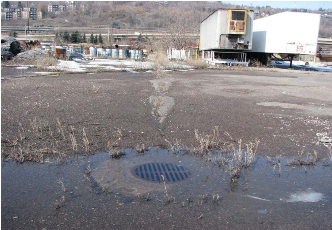
Photo 14 Storm grate inlet in asphalt paved lot area east of former warehouse building.
