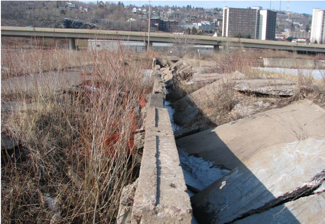
Photo 38 View northwestward of eroded and collapsing dock wall structures near western end of Slip 2. Lot C area to left.
