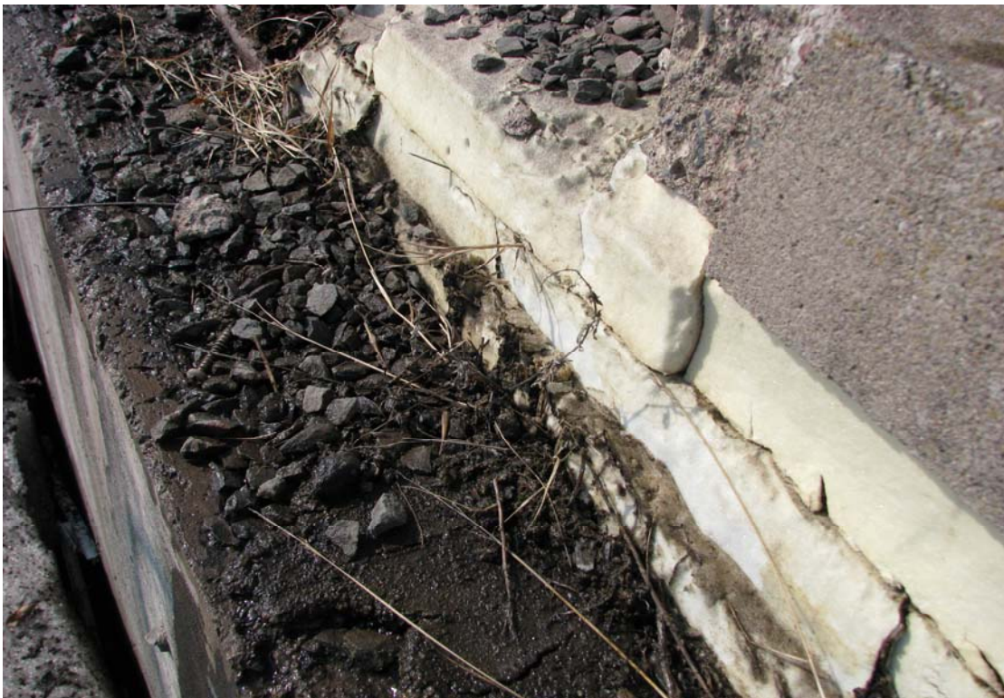
Photo 8 Close-up of foam insulation between former floor slab and foundation slab of former refrigerated warehouse building.
