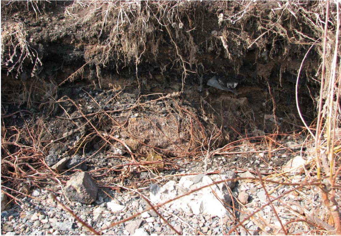
Photo 23 Close-up of eroded fill of Lot D area at southeastern side of Lot beside harbor.
