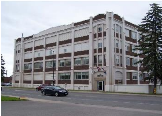
Example of Main Street Building III
