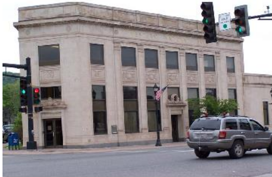
Example of Corridor Building II
