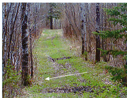
The cross-slope on this trail (arrow) is greater than desired but is not a major issue because it is only for a short distance. If this went on for a distance, skiers would find it annoying.
