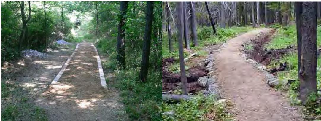
Figure 14: Causeway or Turnpike Trail Construction
