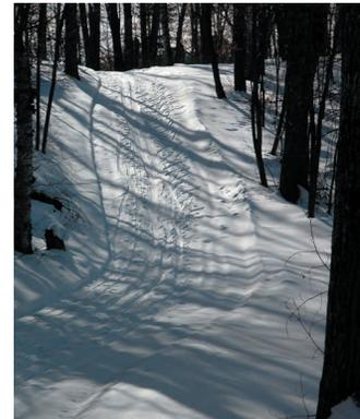
On this steeper uphill section, this two-track traditional trail only widens a foot or two to accommodate herringbone or snowplowing skiers. With light levels of use, there is no reason to make the trail wider on a hill.
