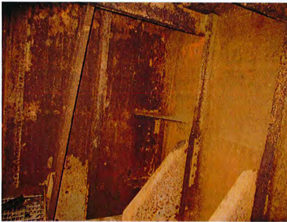
Forward bulkhead to side shell
