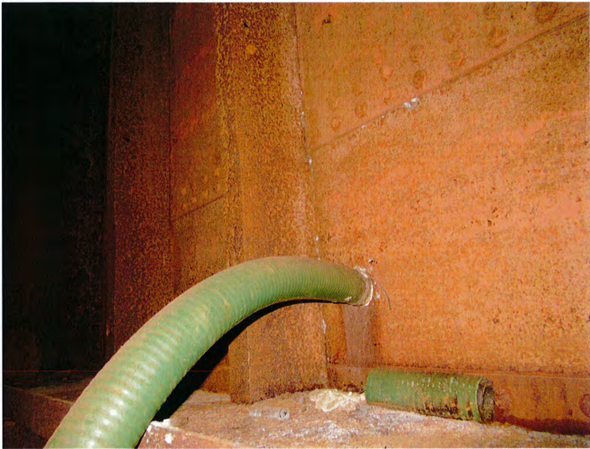
Shell plate access hole
