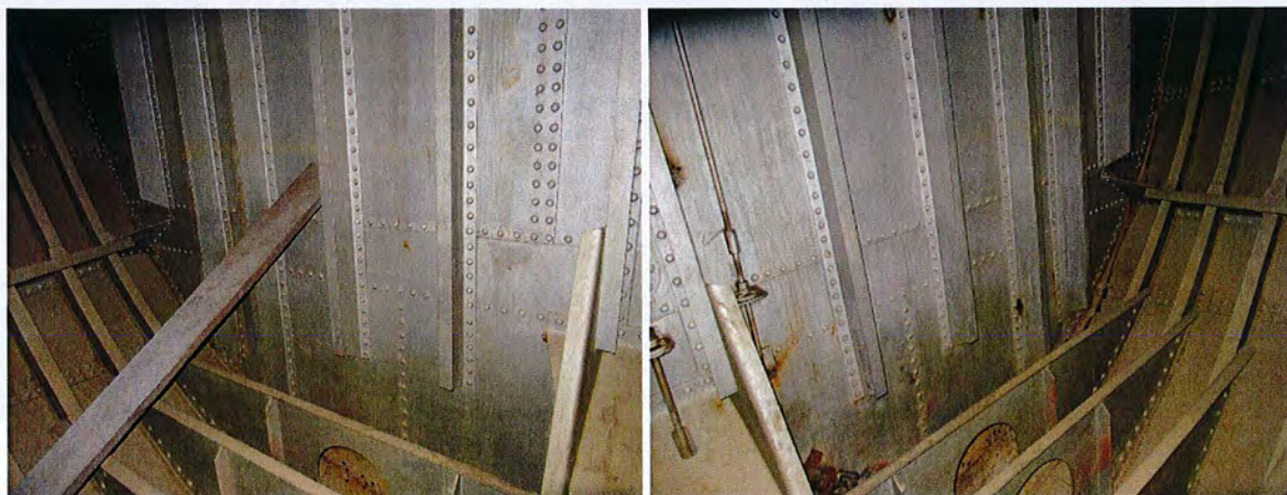
Looking aft – Collision Bulkhead
