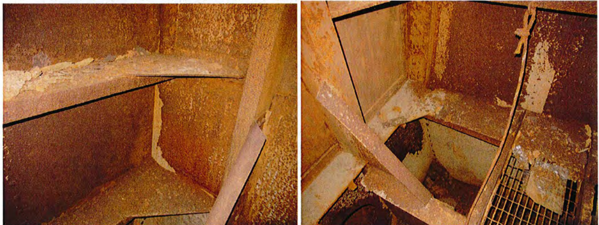
Fore and aft bulkheads
