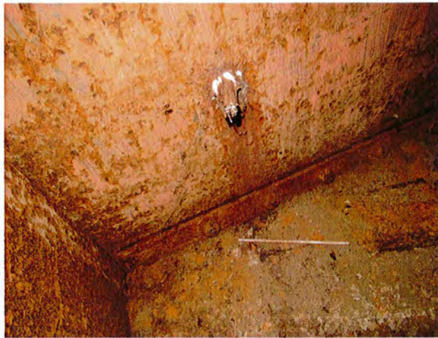
Hole cut through side shell with stick as plug
