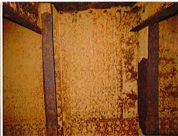
Side shell plating and framing
