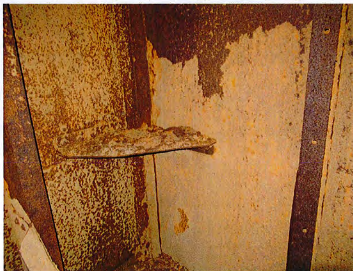
Aft Bulkhead to side shell connection
