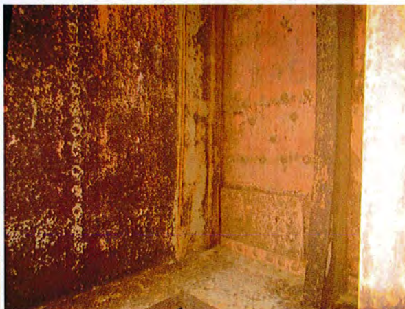
Aft bulkhead to side shell connection
