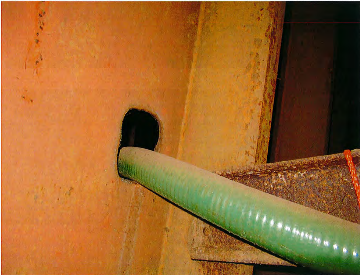
Cargo hold access hole
