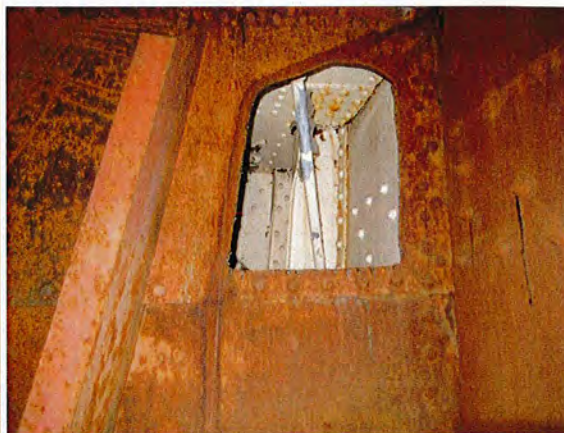
Access hole in forward bulkhead
