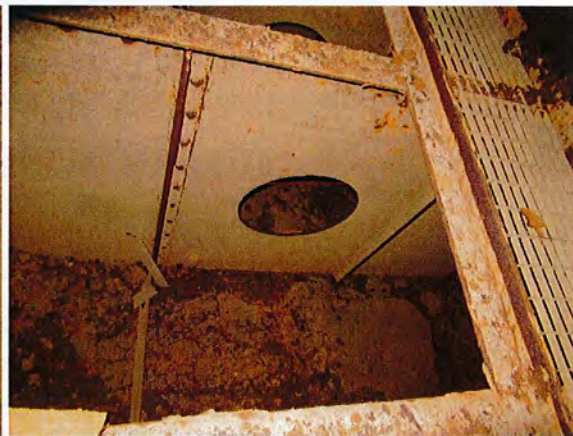
Floor with 22" diameter lightning hole
