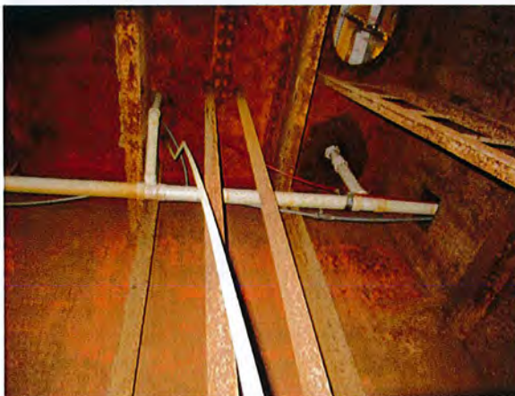
Restroom plumbing and access hole
