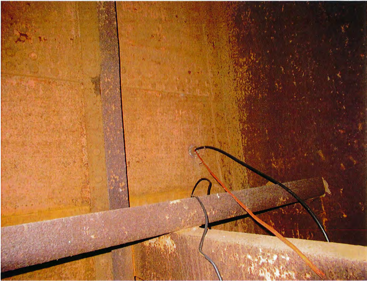
Wiring side shell penetration.
