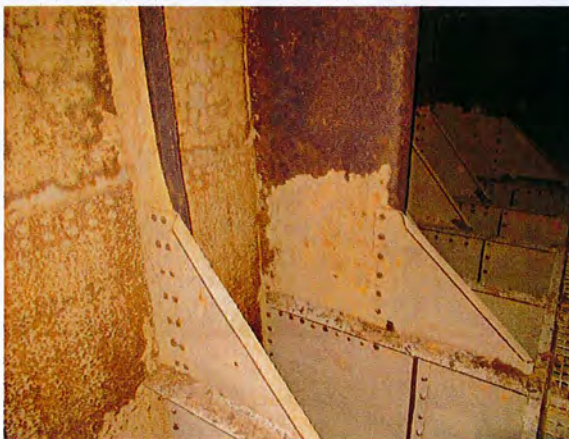
Side shell plating and framing
