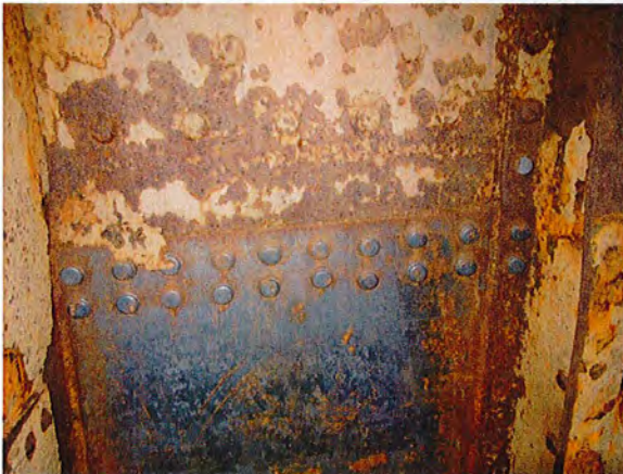
Upper bilge roll (flushed butt)
