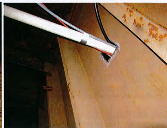
Restroom plumbing and access hole
