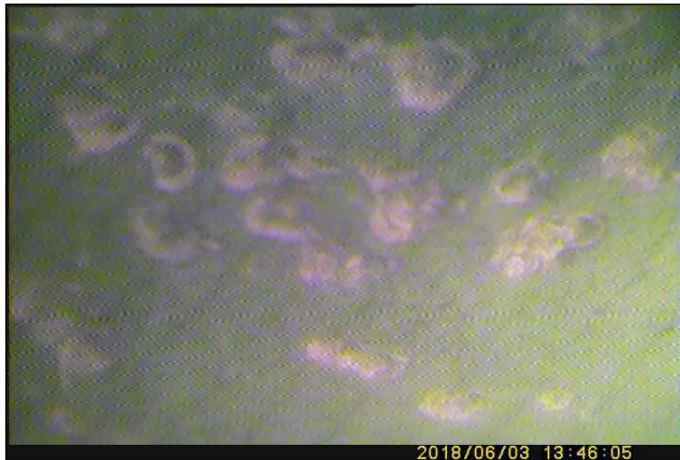
Picture 1: Typical Condition of the Corrosion
