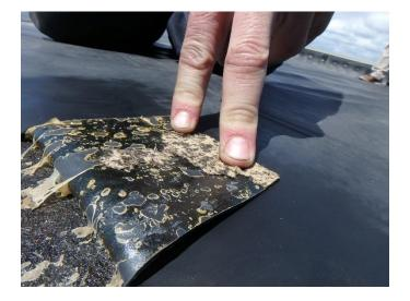
Close up of back side of membrane- note approximately 35% of the adhesive appears to have bonded to the wood fiber cover board.
