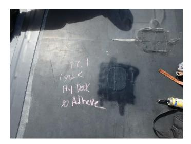
19. Test cut 1 location revealed no adhesion between membrane and plywood substrate. No evidence of moisture intrusion noted.
