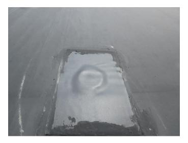
17. Photo documenting typical repair made with plate screwed over the membrane and flashing tape covering.
