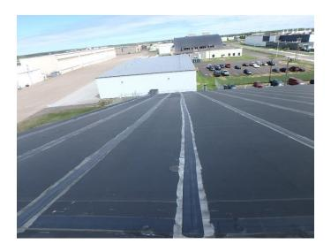
13. East slope. Securement strips have been installed on top of the membrane with flashing tape over the top.
