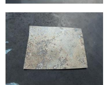
21. Photo documenting back of membrane – little adhesion was ever accomplished between the membrane and plywood. The membrane was completely loose at both test cut locations on Building 2.
