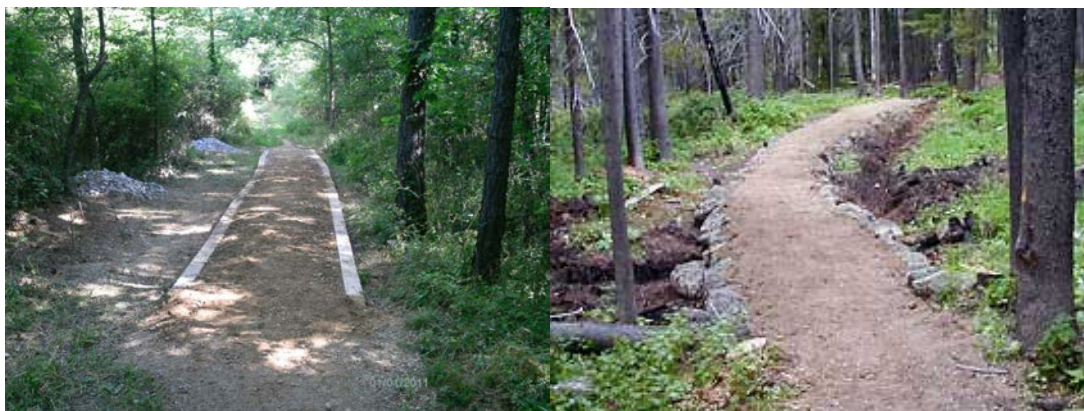
Figure 14: Causeway or Turnpike Trail Construction
