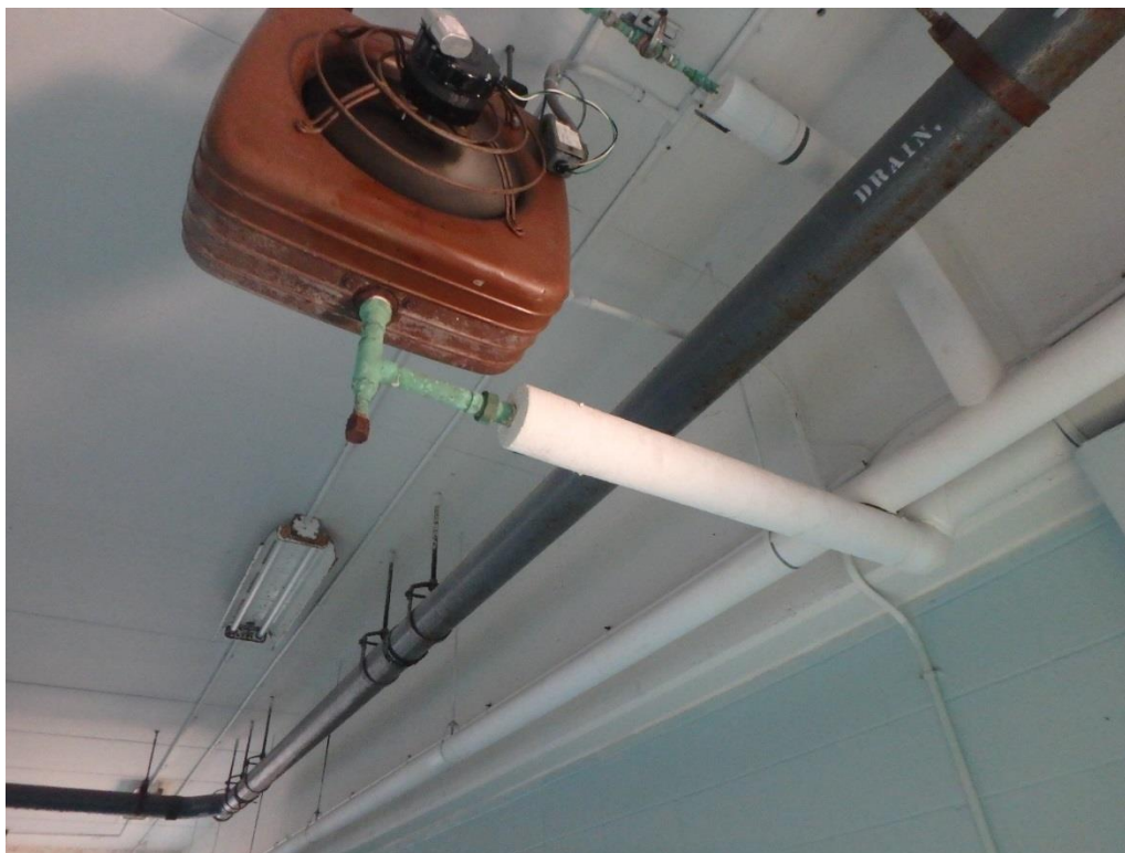
Photograph 1 - Typical unit heater
