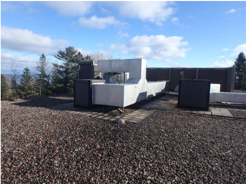
Photograph 4 - Roof top dehumidifier
