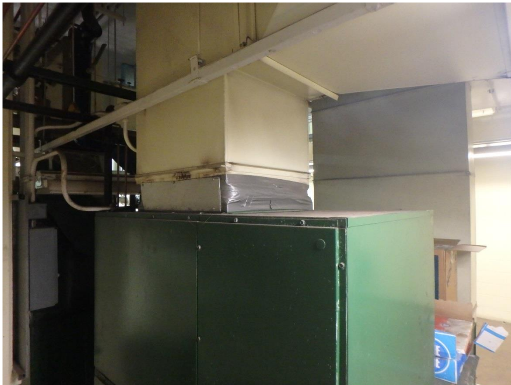
Photograph 2 - Plenum gaskets
