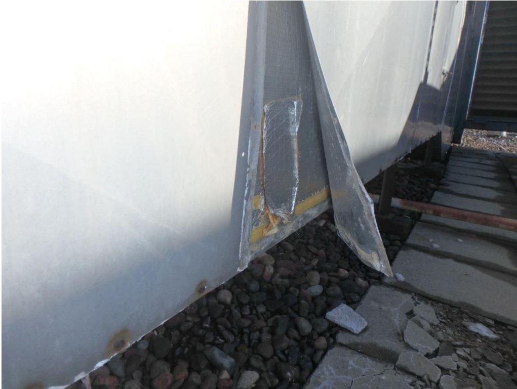
Photograph 5 - Roof top dehumidifier insulation
