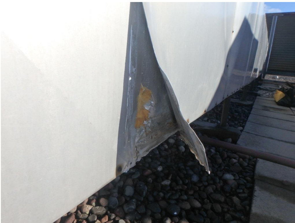
Photograph 6 - Roof top dehumidifier insulation
