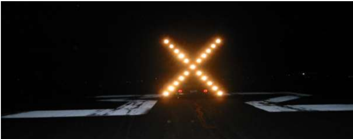
Figure 2-4 Lighted X at Night
