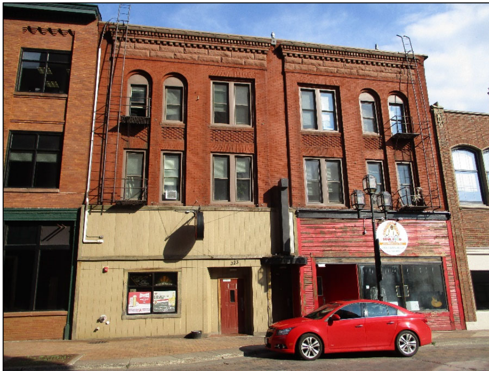
321-323 West 1st Street (Historic Name: Mason Flats)
