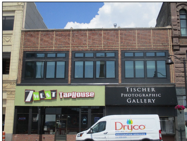
5-7 West Superior Street (Historic Name: Norris-MacDougal Block)
