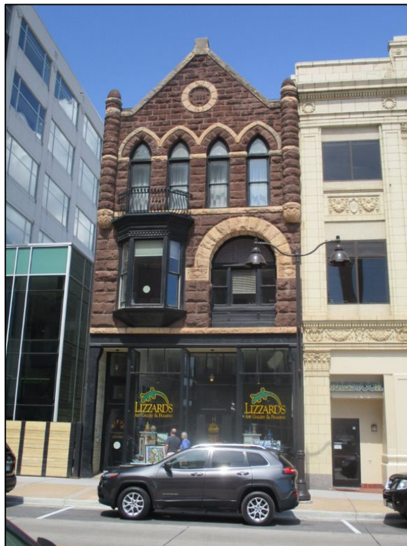
13 West Superior Street (Historic Name: Wirth Building)
