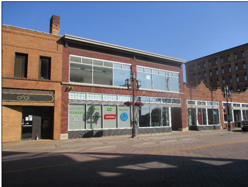
209-211 West 1st Street (Historic Name: Gilbert Building)
