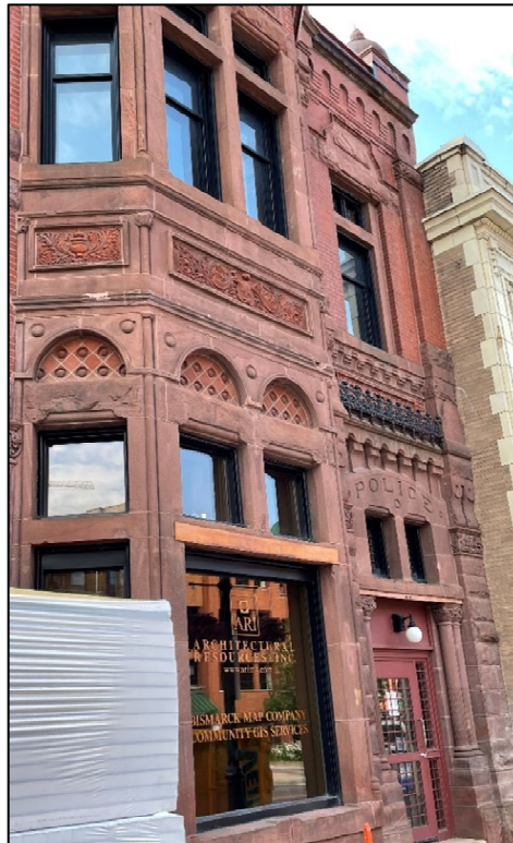
Photograph 17: View of the former Duluth Police Headquarters showing a variety of decorative architectural features including cast iron railing, molded brick and brick corbels, and carved stone.
