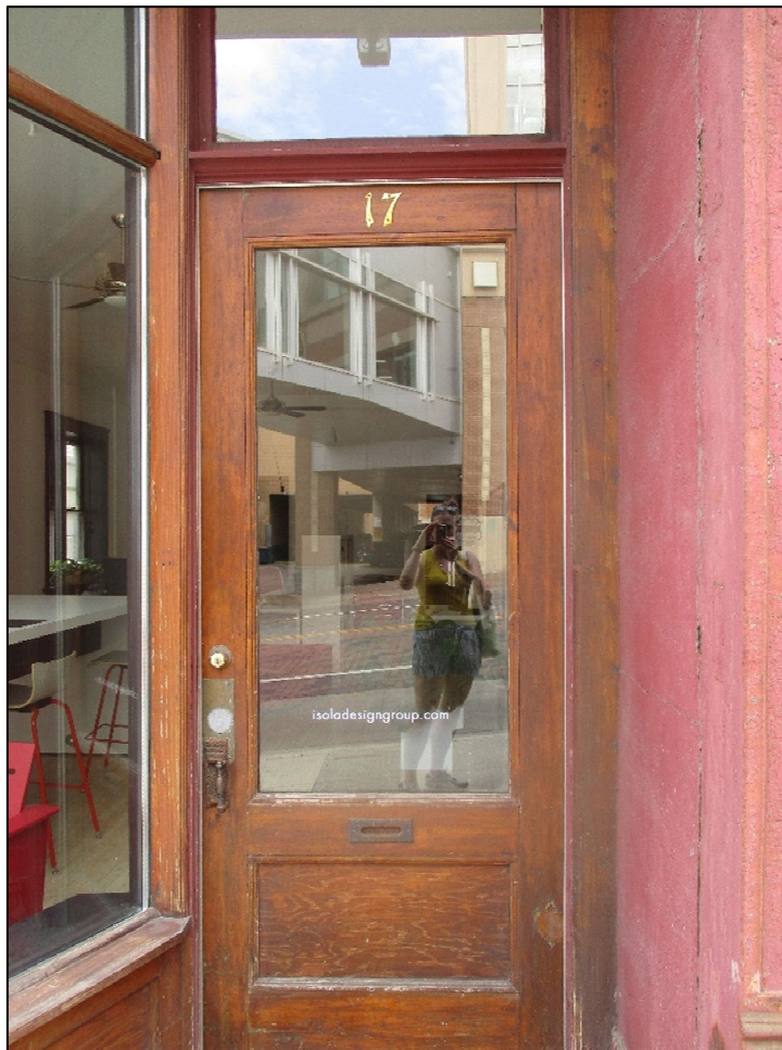
Photograph 16: View of a typical historic wood panel door in a commercial storefront with some of its original hardware.
