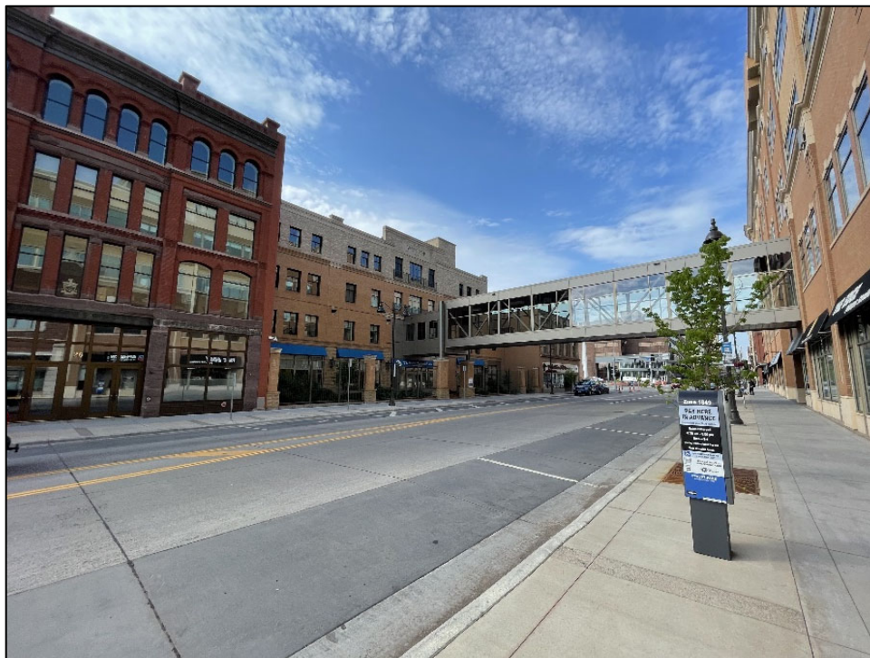
16-24 East Superior Street (Non-historic infill)
