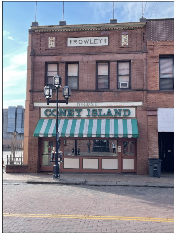
112 West 1st Street (Historic Name: Rowley Building)
