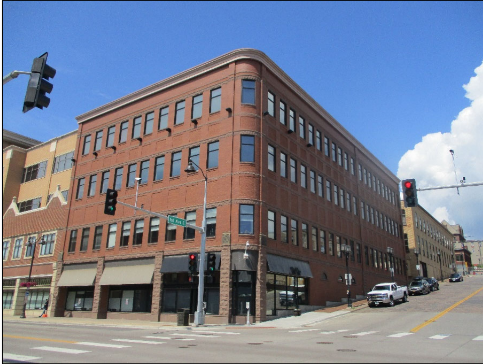
13 East Superior Street (Non-historic infill)
