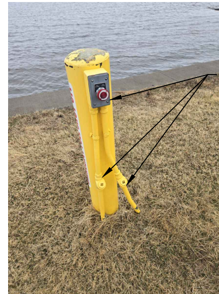
EXISTING EMERGENCY SHUT OFF PEDESTAL NOT TO SCALE
