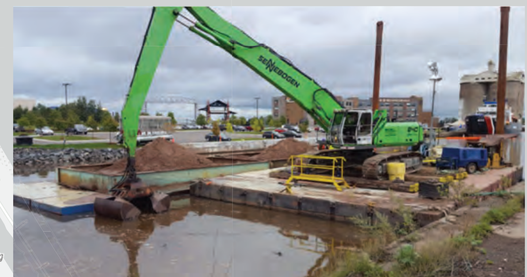
Capping Contaminants in Slip 3, 2018
