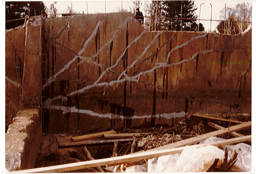
#11 10/16/85 FACE OF SOUTH WALL AFTER INJECTION
