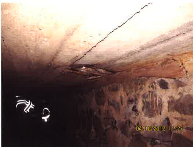
Photo 9A (19+75) – Hole in Roof & Poor Masonry
