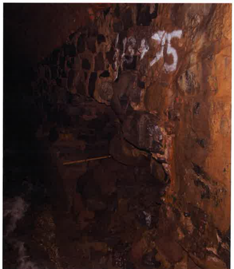
Photo 1B & 1C (Station 13+75) –Sect. 1 Bulge and Voids in Wall Before (4/11) and After (6/29) the Flood
