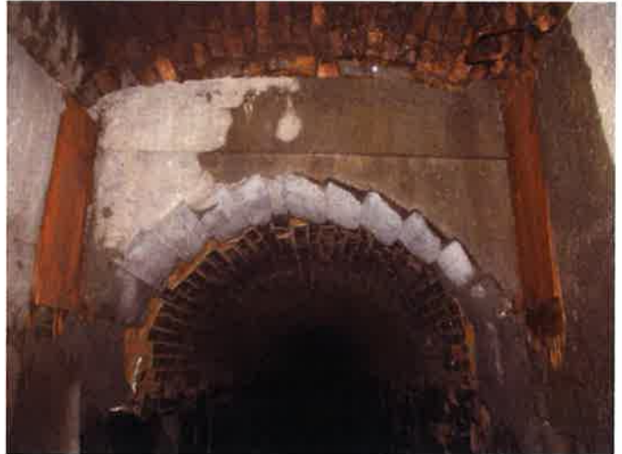
Photo 1D & 1E (Station 11+00) – Manhole Failure Before and After Repair
