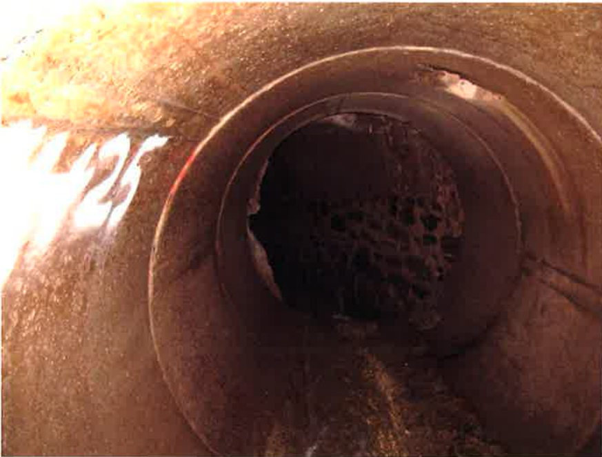
Photo 2A & 2B (Station 14+25) –General Condition of Section 2 (A) and Eroded Floor Invert (B)
