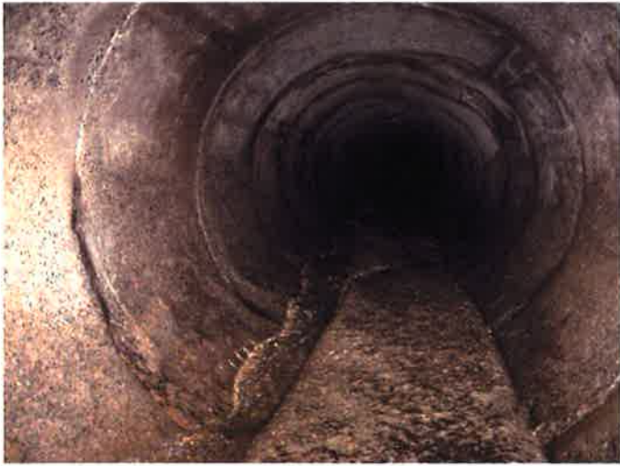
Photo 29A (47+45) – Eroded Invert and B/Pipe
