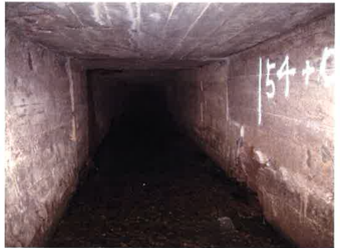
Photo 34C (54+00) – General Condition and Sagged Roof
