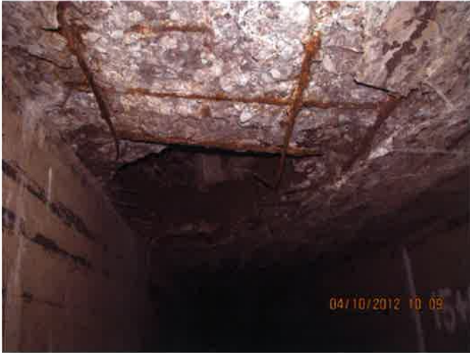
Photo 3A (14+95) – Roof Failure (Relaced Sum. 2012)
