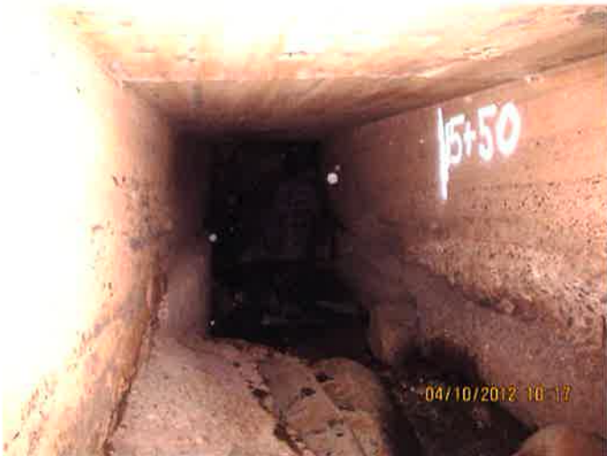
Photo 3C (15+40 to 15+75) - Scour in wall & Underpin
