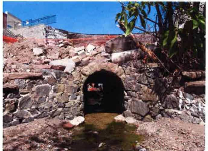
Photo 11A (23+57) – Deteriorated Headwall
