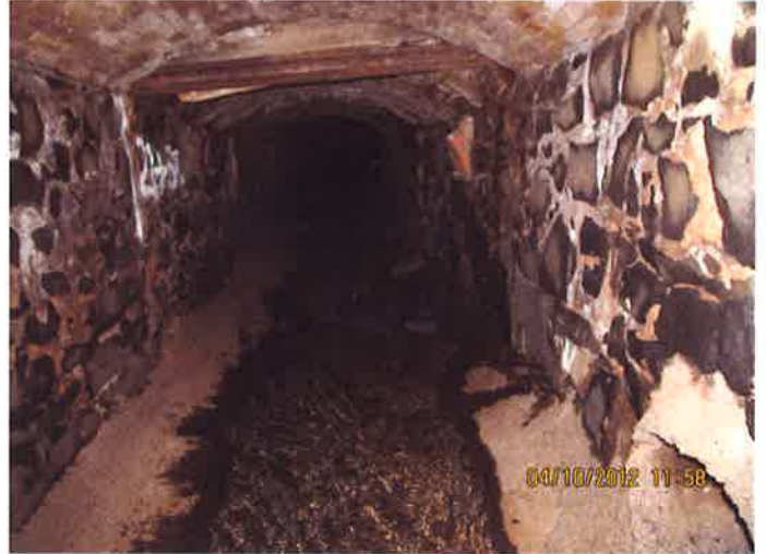
Photo 10C (21+50) – Corroded Support Beam in Roof
