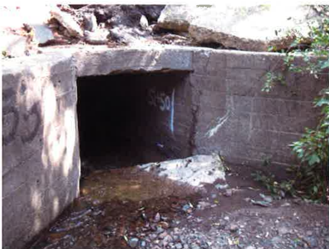
Photo 32C (51+51) – Debris at Inlet
