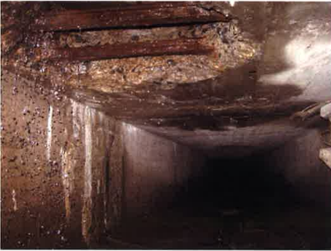
Photo 20C (34+25) – Roof Failure @ Manhole
