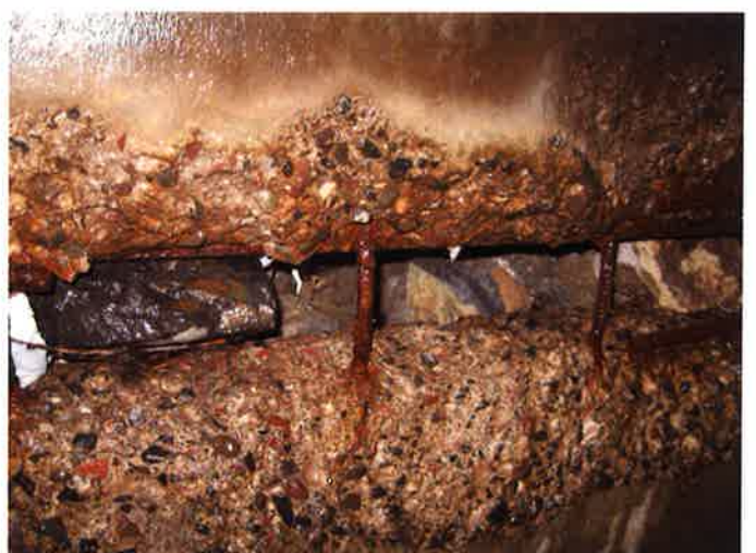
Photo 14B (Sta 27+00) - Hole in Roof
