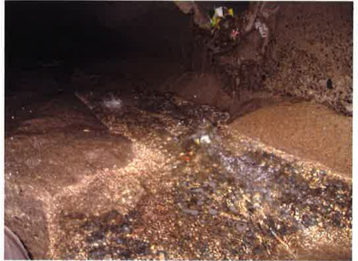
Photo 20B (34+25) – Floor Failure
