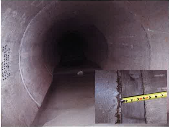
Photo 12B (25+00) – Condition & RCP Joints
