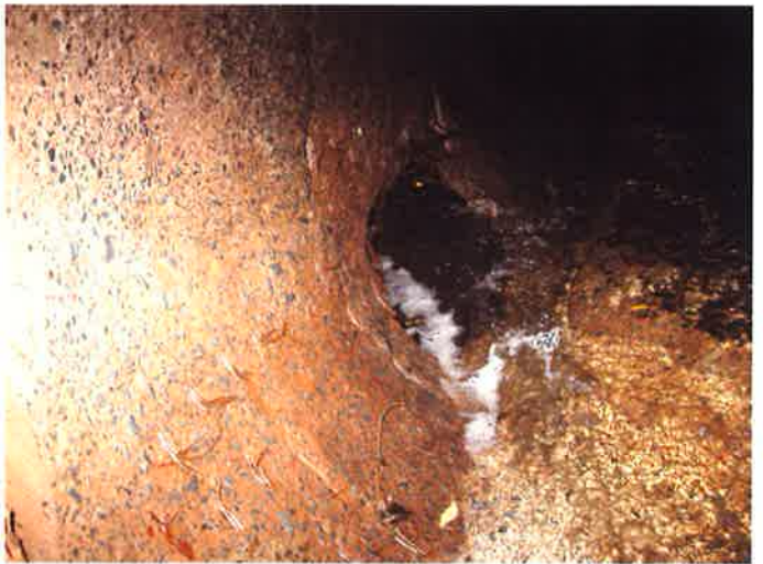
Photo 29B (47+35) – Hole in pipe @ Flow Line
