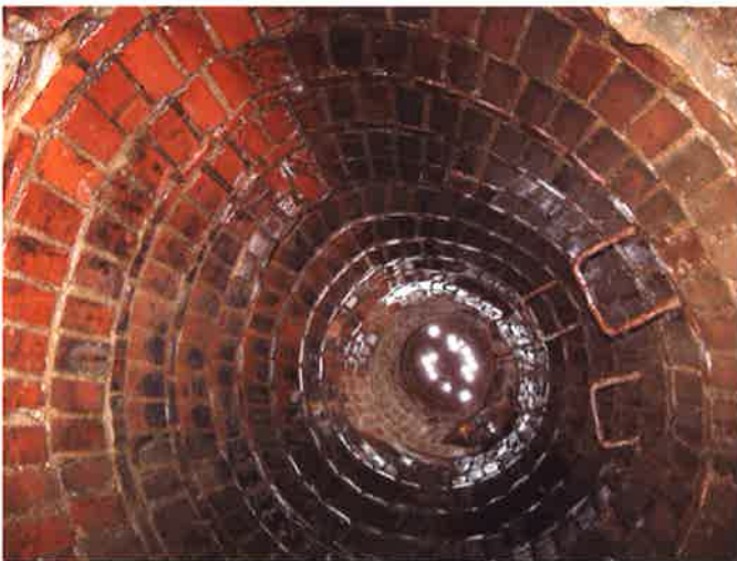
Photo 18B (30+13) – Bulged Manhole Riser
