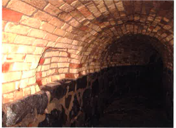
Photo 16A (27+75) – Eroded Brick Roof
