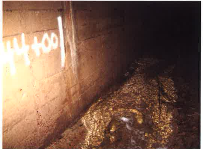
Photo 28B (44+00) – Failure of Floor
