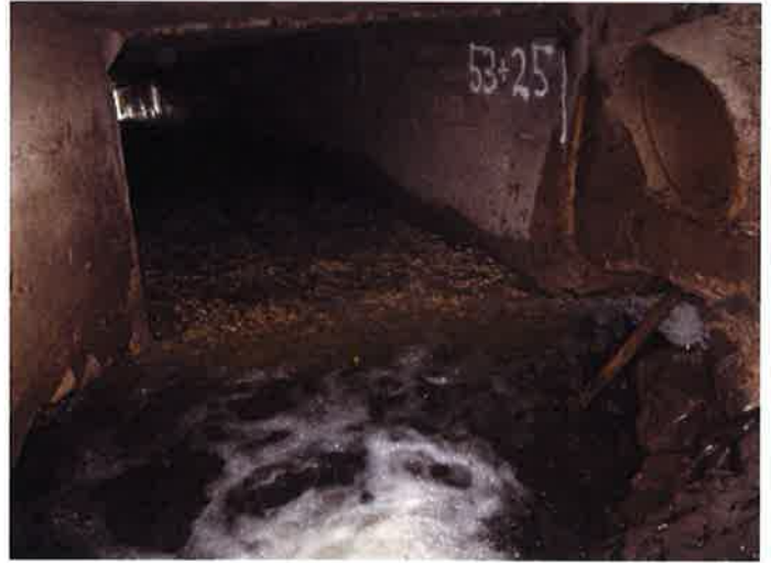
Photo 34A (53+25 – 53+34) – Floor Failure
