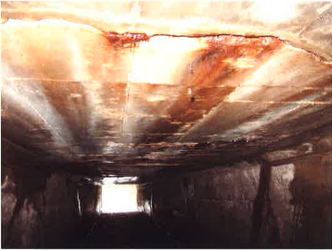
Photo 33B (52+70) – Exposed Bar and Cracking in Roof
