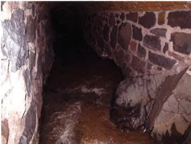
Photo 10D (22+48) – 4’ Scour in South Wall (6/29)
