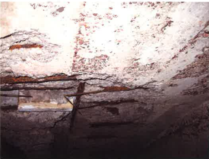
Photo 21A (37+40) – Spall in Roof
