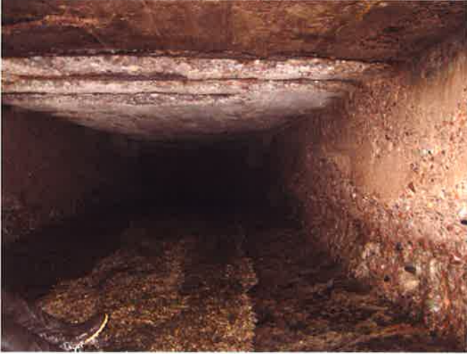
Photo 20A (32+25) – Roof & Wall Spalling
