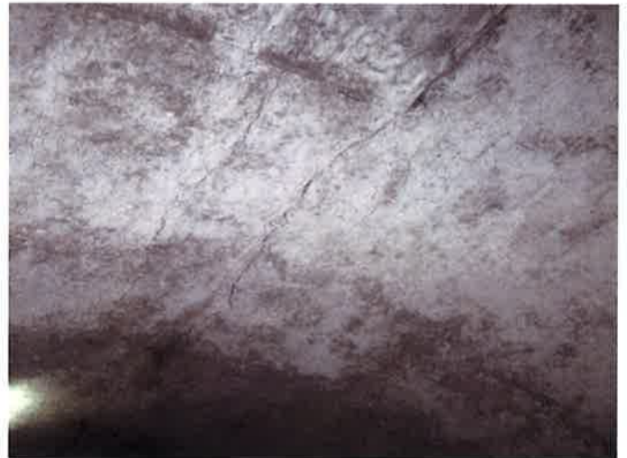
Photo 31B (48+75) – Cracking of RCP Roof
