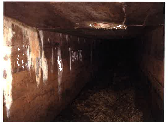
Photo 19A (30+75) – Cracked and Sagging Roof
