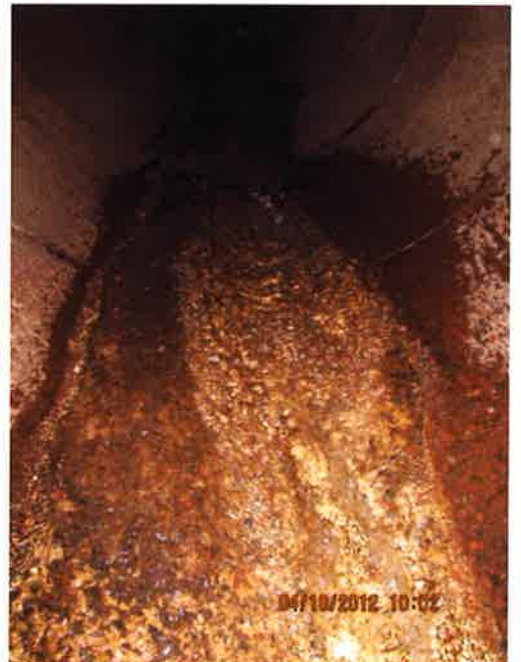
Photo 2A & 2B (Station 14+25) –General Condition of Section 2 (A) and Eroded Floor Invert (B)
