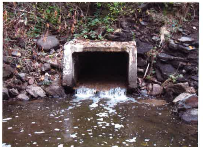
Photo 33A (52+08) – Outlet with Failing Floor
