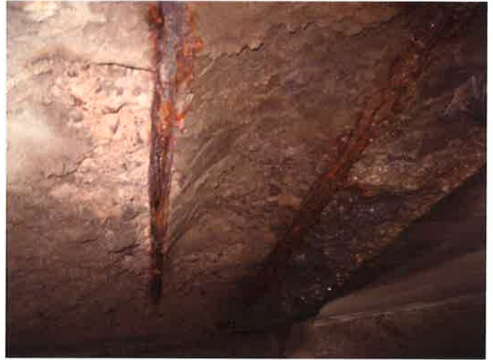
Photo 20D (35+35) - Severe Spalling of Roof
