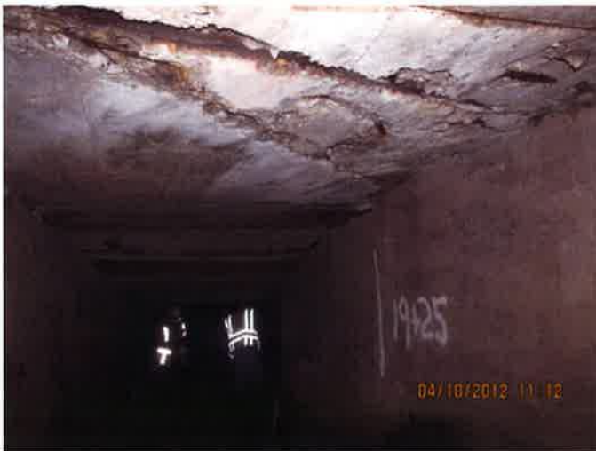
Photo 8A (19+25) – Failing Roof
