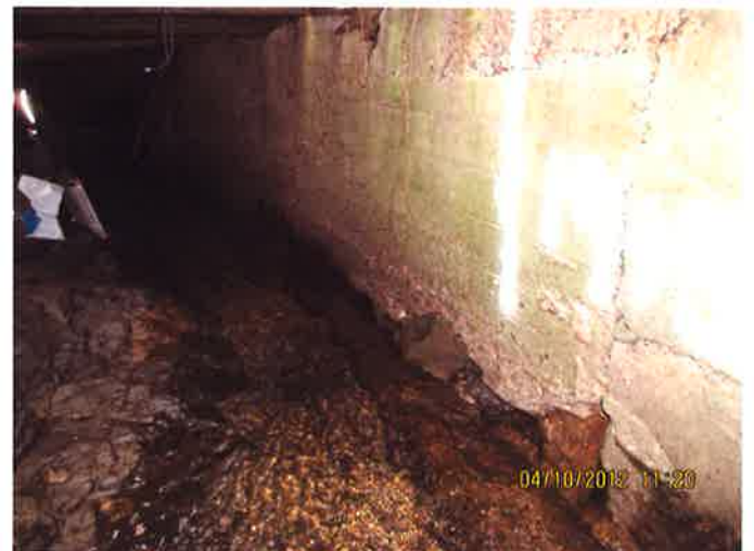
Photo 8B (19+50) – Scour at Bottom of Wall
