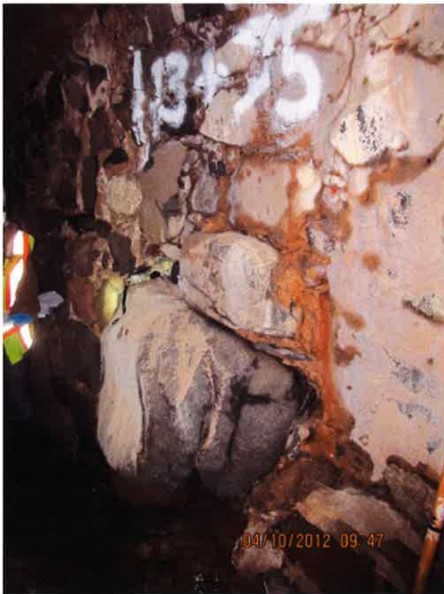
Photo 1B & 1C (Station 13+75) –Sect. 1 Bulge and Voids in Wall Before (4/11) and After (6/29) the Flood
