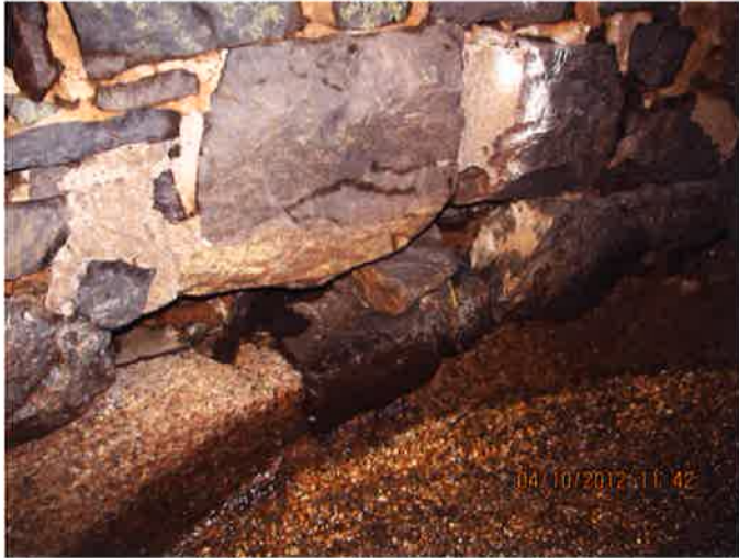
Photo 10B (20+60) – Scour of Lower 18” of Wall
