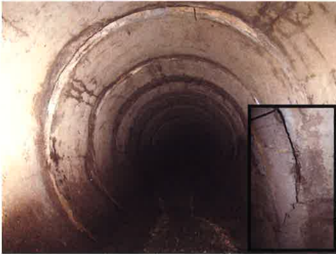
Photo 31A (49+50) – Gen. Cond. & Separated Joint
