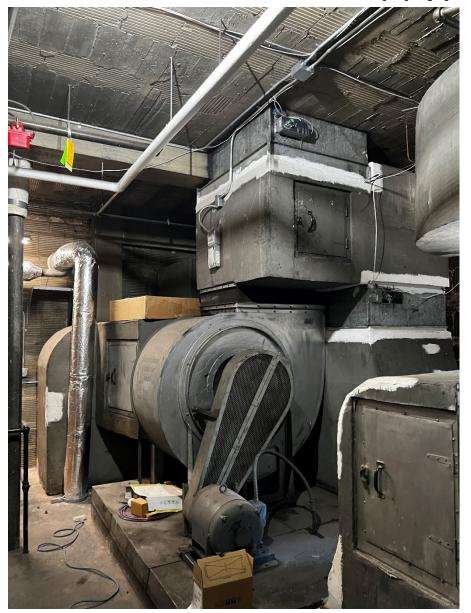
Current ventilation system does not meet OSHA or MN Depart of Health guidelines for air quality. Existing system is grandfathered in. Existing system is original equipment from 1927, almost 100 years old.
