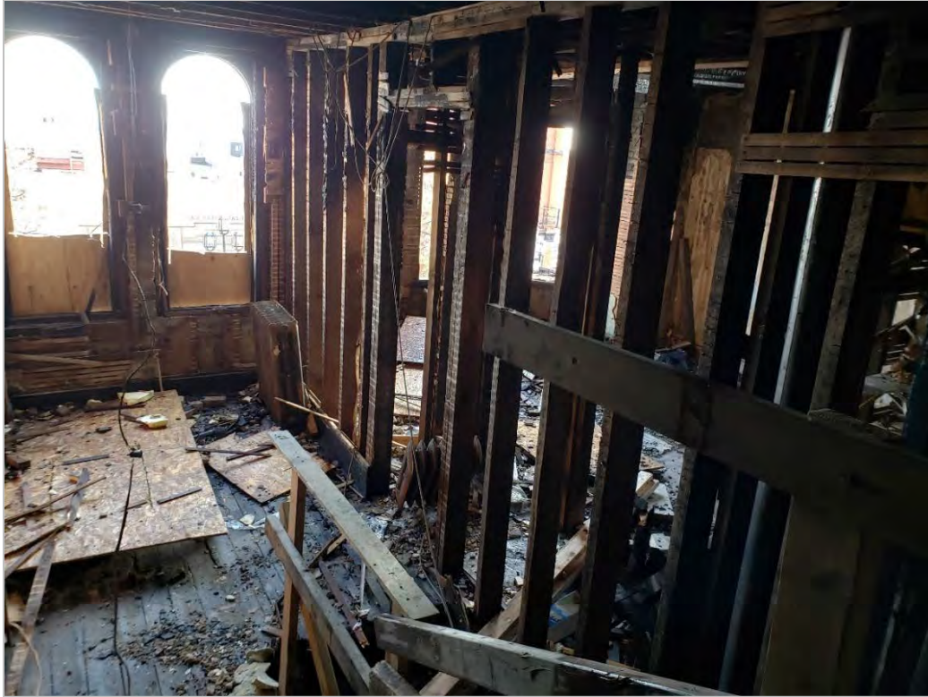
Photo 11: Pastoret Building easterly module, Level 2 looking south. Random direct fire damage this level and extensive water infiltration.
