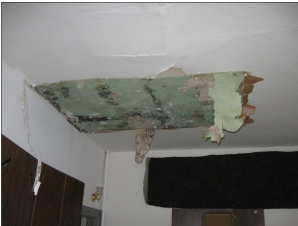
Figure 9 Typical interior of upper level ceilings showing sporadic water damage
