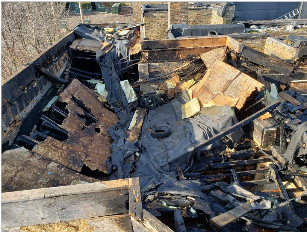
Photo 4: Close up view of fire destroyed and collapsed roof system of Pastoret Building westerly module.
