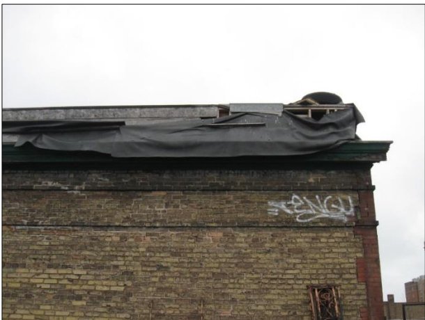
Figure 19 Southwest corner of Pastoret Terrace showing deteriorated temporary roof over burn areas
