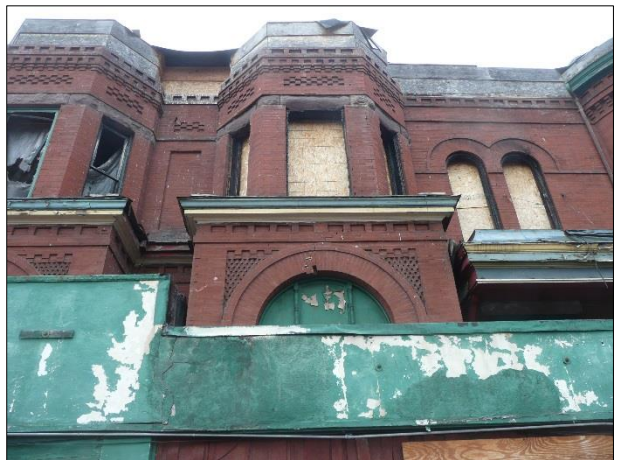
Figure 26 Loose brick at window arch, brick needs to be tuck-pointed
