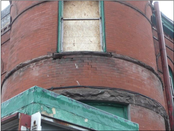
Figure 23 Loose Sandstone band, stair step crack, brick needs to be tuck-pointed
