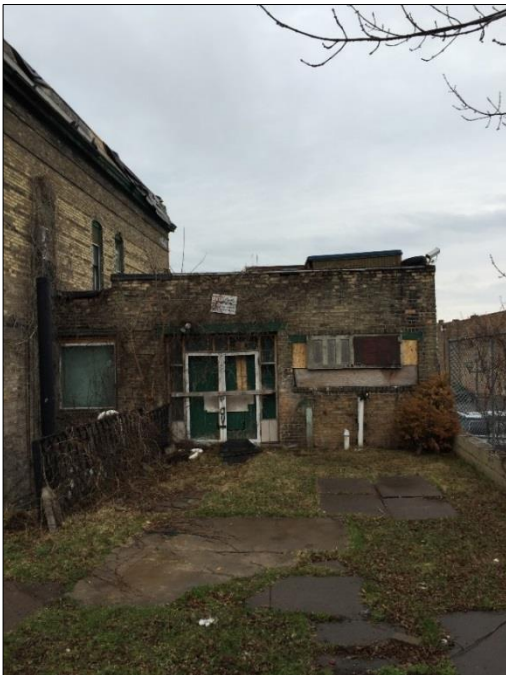
Figure 39 Rear of Paul Robeson Ballroom, Brick needs to be tuck-pointed, parapets need to be repaired
