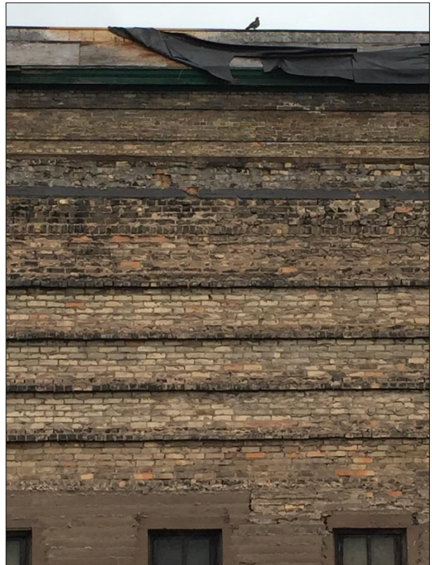
Figure 36 Side of Paul Robeson Ballroom, Damaged brick, brick needs to be tuck-pointed, parapet needs to be repaired
