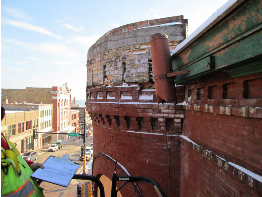
Photo 19: Upper wall region, east elevation looking south. Substantial efflorescence, loss of pointing mortar and loose bricks.
