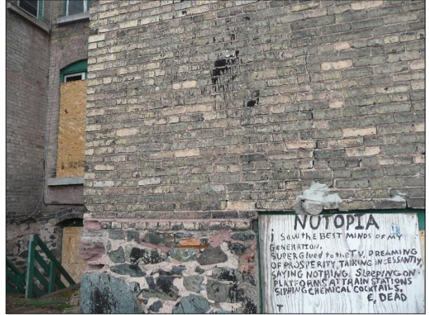
Figure 30 Brick on rear of Pastoret building needs to be tuck-pointed
