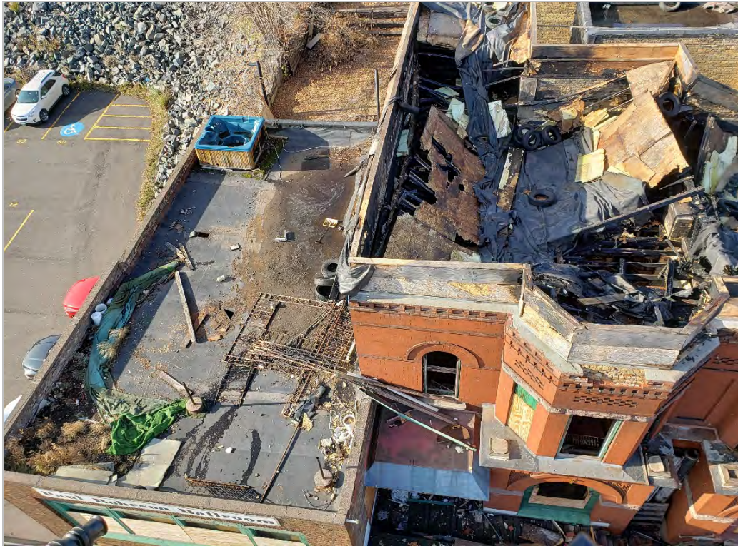
Photo 7: Robeson Building roof (left side of photo). Initial assessment indicates fire damage from recent fire may be confined to region directly adjacent to Pastoret Building west wall, but water saturation was identified throughout interior.
