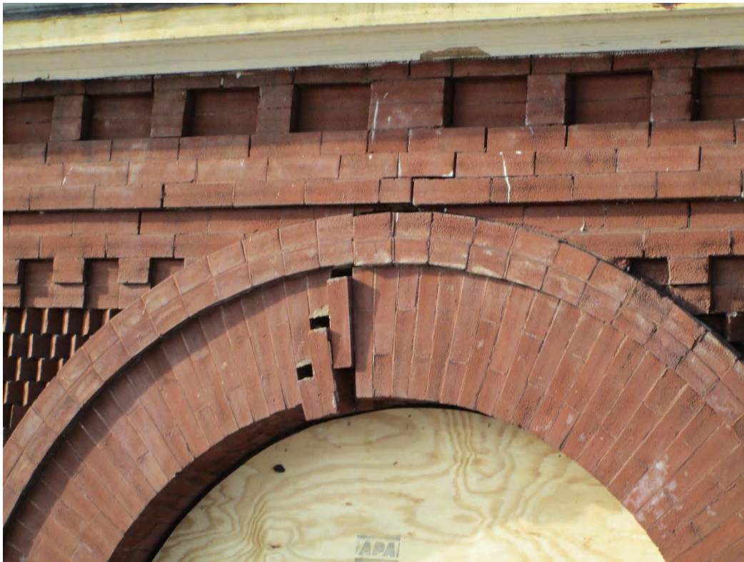
Photo 24: Typical brick displacement/failure at arched window header, Level 2, south elevation (easterly module shown, westerly module similar).
