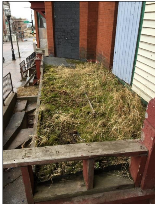
Figure 40 Vegetation growing on low roof, deteriorated roof structure below
