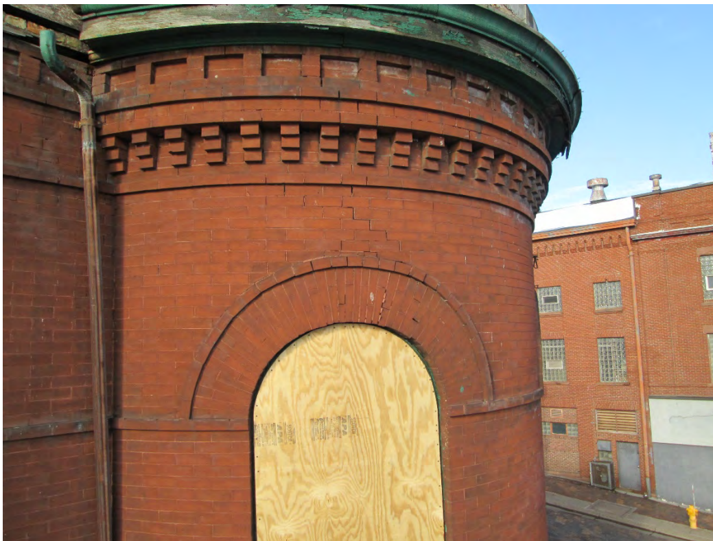
Photo 22: Southeast corner turret., south face. Joint cracking and brick end gap openings above window indicate potential global movement in wall circumference brick.
