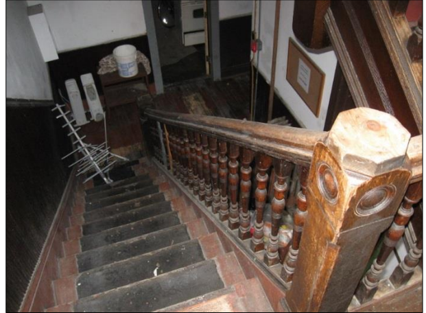
Figure 8 Example of interior wood stairs that can be retained serving second floor
