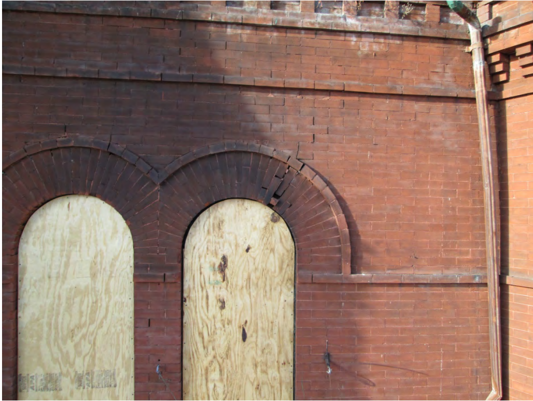
Photo 23: Typical brick displacement/failure at arched window headers. Level 3, south elevation, easterly module adjacent to southeast corner turret.
