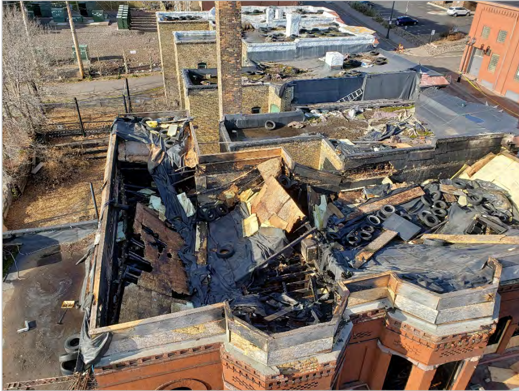
Photo 3: Fire destroyed and collapsed roof system of Pastoret Building westerly module.
