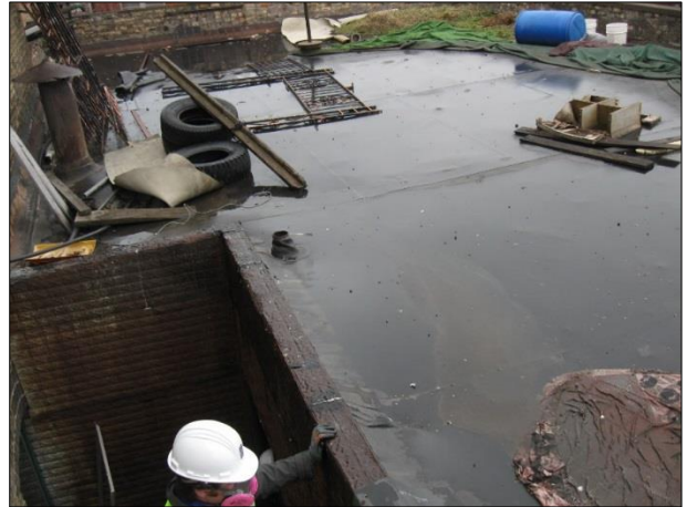
Figure 18 EPDM roof over Ballroom area. Note growth in corner and debris.
