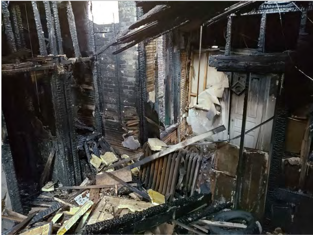
Photo 9: Looking into Level 2 of Pastoret Building westerly module from northeast corner region of 2 nd floor level of Robeson Building. Interior walls and framing are entirely compromised. Heating radiators are presently unsupported/ collapsing through floor.
