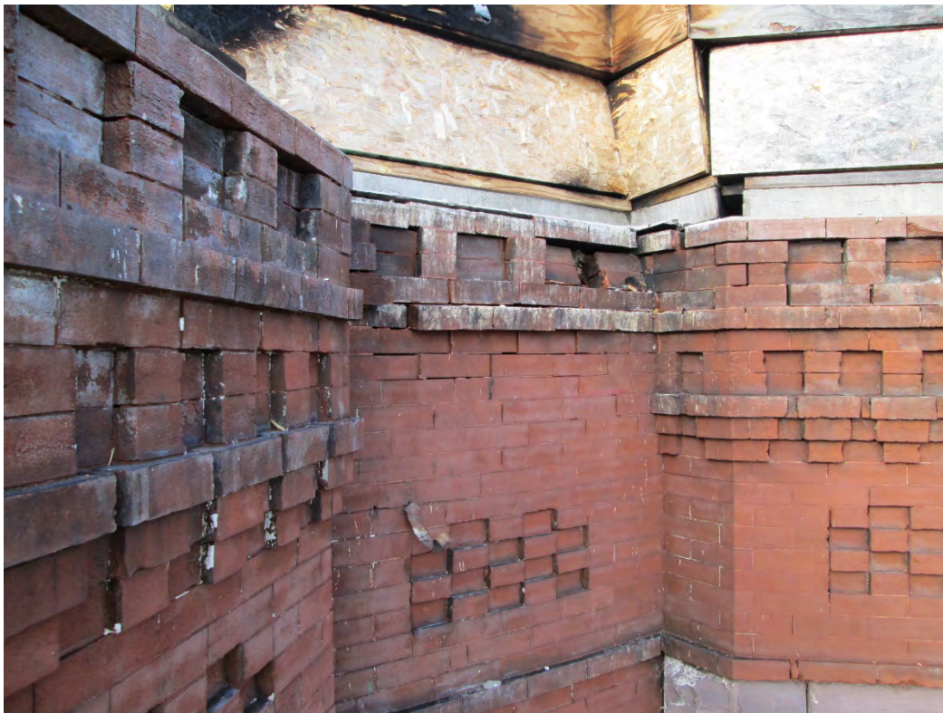
Photo 14: Closer view from previous photo. Looking east, upper region, brick displacement/loose brick, significant efflorescence and loss of pointing mortar.
