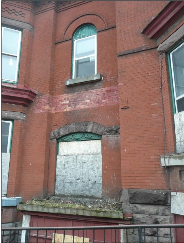
Figure 27 Mismatched brick, existing brick needs to be tuck-pointed
