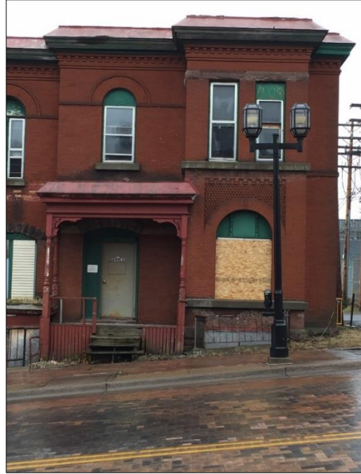
Figure 38 Entry stairs need to be replaced. Wrought iron railing needs to be repaired or replaced.
