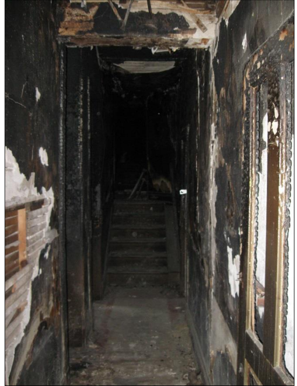
Figure 12 Corridor leading up the hill to serve inside units. Fire and smoke damage from front end fire
