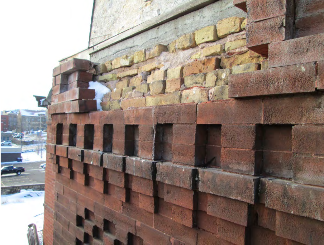
Photo 17: Close up of devoid brick area from previous photo. Numerous loose bricks remain and present a hazard to below.
