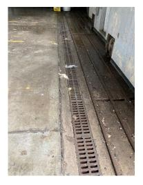
Bituminous pavement shall be placed over the door tracks. The trench drain shall be sealed and capped to the best of the contractor's ability and paved over with bituminous pavement.
